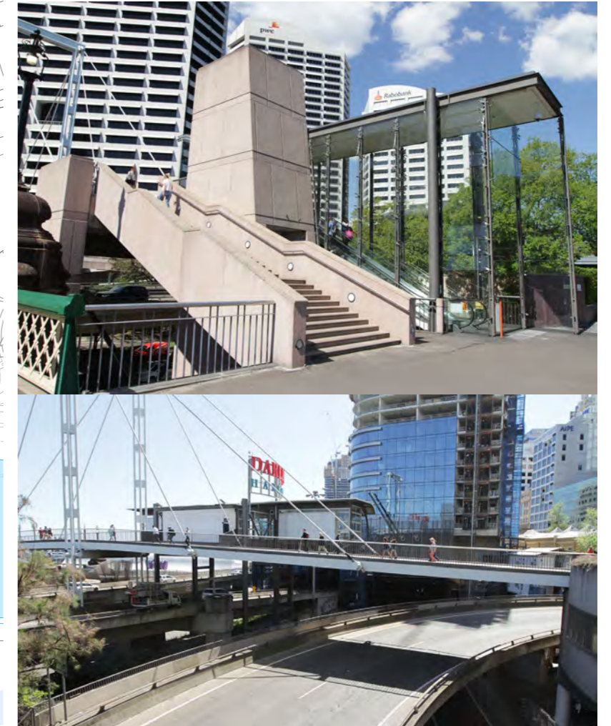
Fig. 52. Existing Pyrmont Bridge connection
