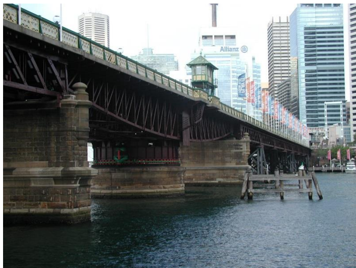
Figure 8 – Pyrmont Bridge viewed from the south west Source: JBA
