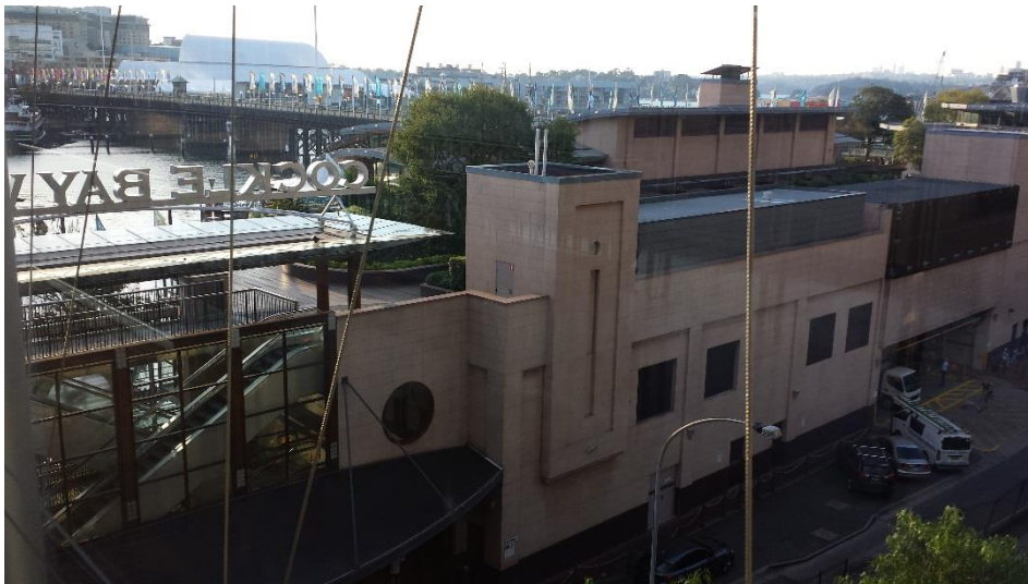
Figure 5 – Rear of current development viewed from the Darling Park foot bridge Source: JBA
