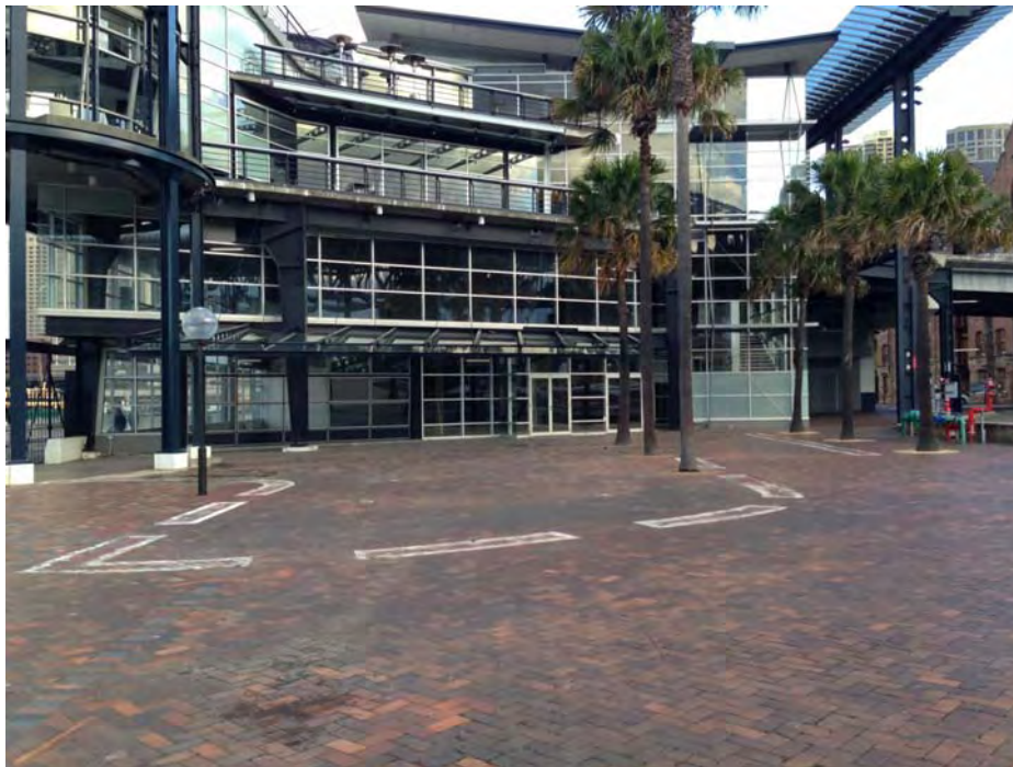
Photograph 2.2 Northern end of OPT - white marking show extent of lease (4 August 2016)
