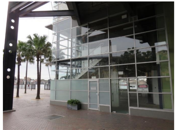
Figure 3.10 Tenancy 5 west elevation. (Source: GML July 2016)
