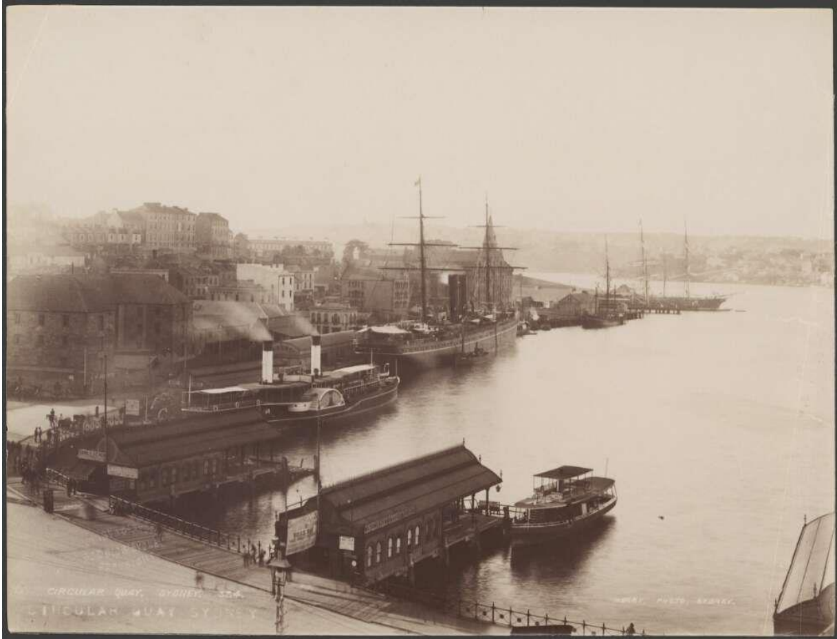
Figure 2.3 Sydney Cove's western shore in 1895, showing the Commissariat Store on the left. The ASN Co. Building can be seen behind a ship's mast. (Source: National Library of Australia < http://nla.gov.au/nla.obj-141606290 >, viewed 8 August 2016. Photographer: Charles H Kerry)
