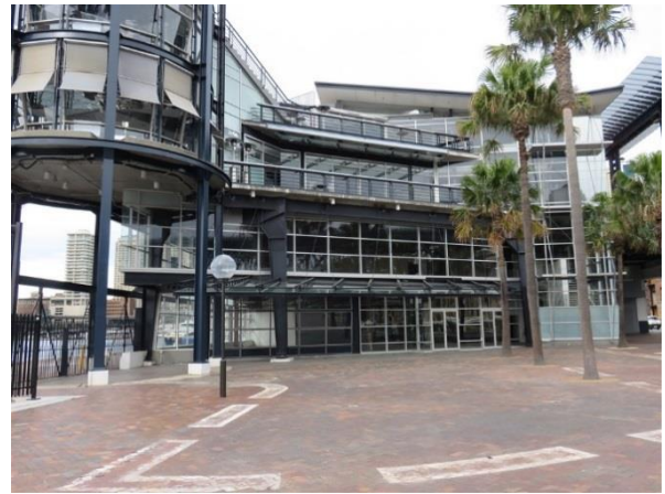
Figure 3.8 The north elevation of the OPT, with the northern outdoor area of Tenancy 5 in the foreground. (Source: GML July 2016)
