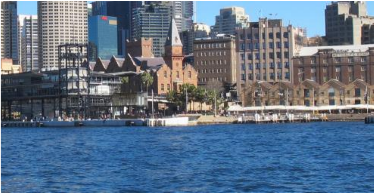
Figure 6.3 Photomontage showing the effect of the brewery pod on views of the ASN Co Building from Sydney Harbour to the northeast of the OPT. (Source: Collins and Turner, 257_ADA_088B)
