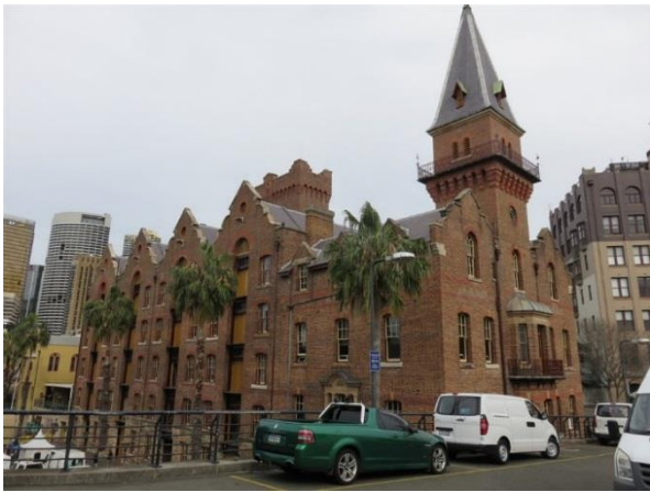
Figure 3.14 The ASN Co. Building, as seen from the northwest. In the foreground is the raised roadway connecting to level 3 of the OPT. (Source: GML July 2016)
