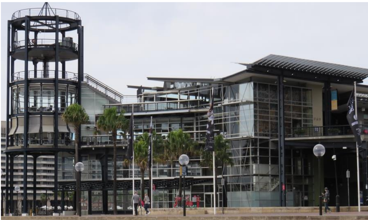
Figure 3.6 The OPT from the northwest. Tenancy 5 includes the two lower floors plus the outdoor area in the foreground. (Source: GML July 2016)
