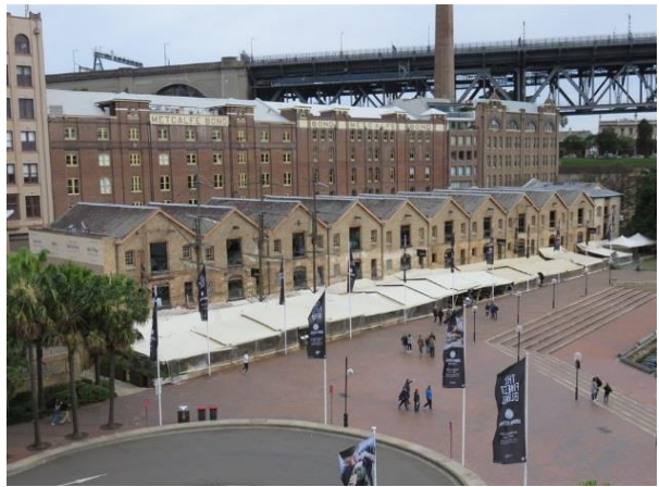
Figure 3.15 Campbell's Stores, as seen from the northeast. (Source: GML May 2016)
