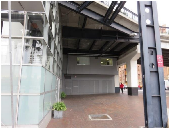
Figure 3.9 The paved area to the west of Tenancy 5. The raised roadway over can be seen over part of the area. The western deck is proposed to be located here. (Source: GML July 2016)
