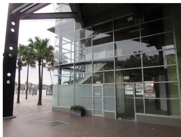
Figure 3.10 Tenancy 5 west elevation. (Source: GML July 2016)
