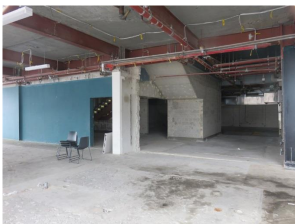
Figure 3.11 Existing internal condition, Tenancy 5. (Source: GML July 2016)
