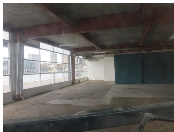
Figure 3.12 Existing internal condition, Tenancy 5. (Source: GML July 2016)
