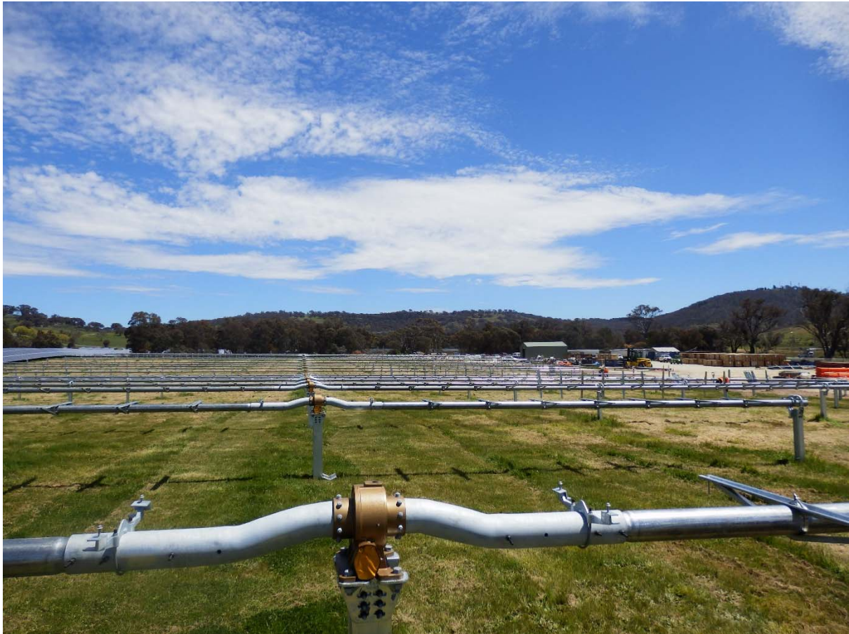
Figure 3-8 Tracker Frames at Mugga Lane Solar Park
