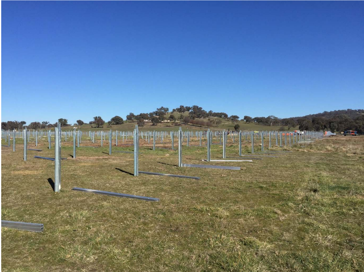
Figure 3-7 Tracking Piles
