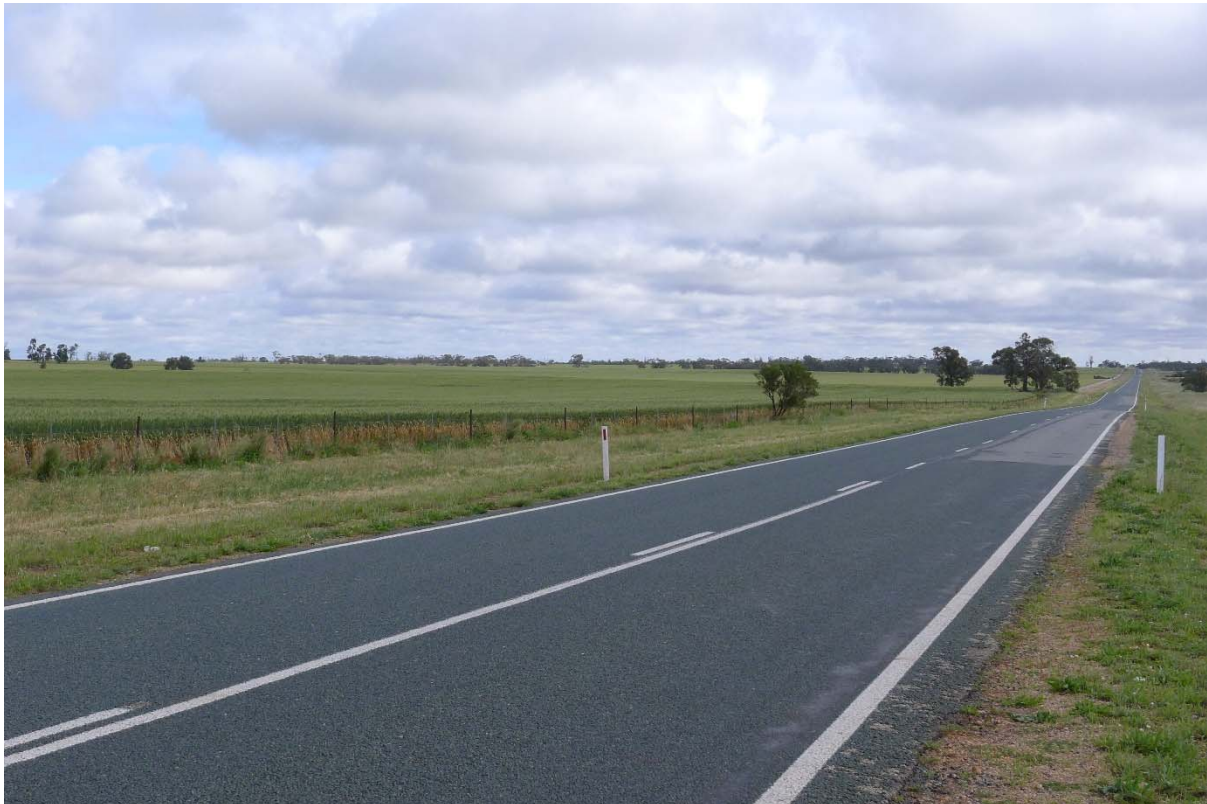
Figure 3-4 View of Balranald-Tooleybuc Road looking north
