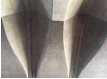
CEILING FINISH XC - Existing pre-form concrete beams.
