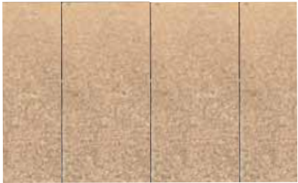
XPC2 - Existing precast granite wall Panels (Cleaned and lightened)
