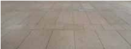
TPC1 - New GRC (Glass reinforced concrete) pre-cast floor tile to Lift 1 and Lift 36 Corridor to match existing Western Foyer tile.
