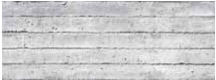
XPCS - Existing Boarded Precast Concrete Strutural Walls Painted
