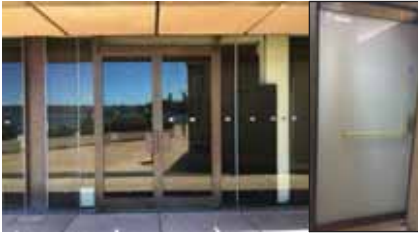
DOORS XGLBF - North Wall Bronze framed double door, hinged entry door XFGL - Existing frosted glazing. Bathroom hinged doors
