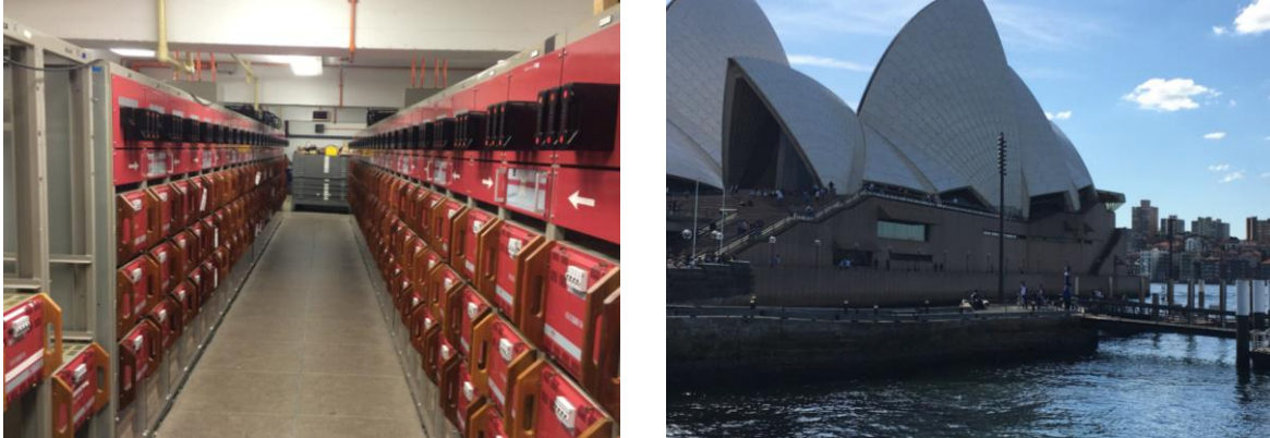
Figure 12: Existing plant room on eastern side of building (left) and view to eastern facade (right) (source: KEYLAN)
