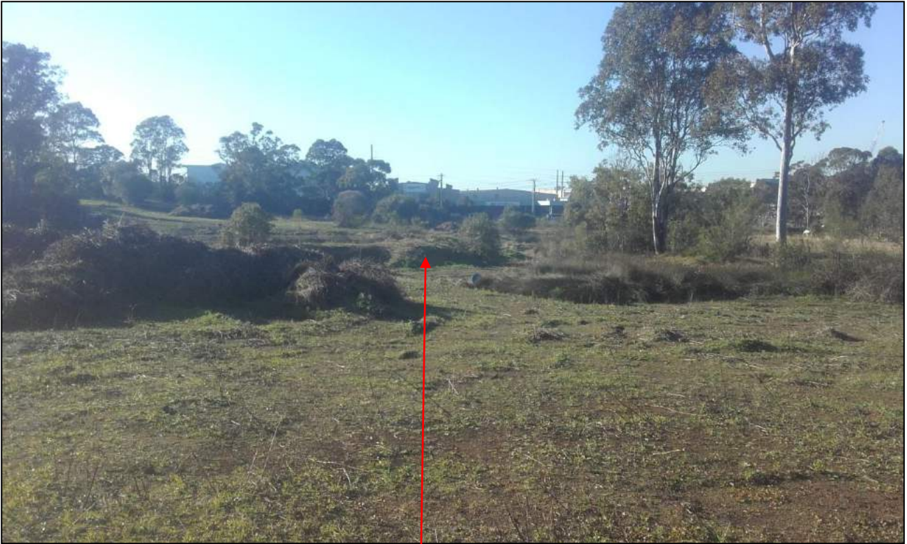
Photograph 9 – Lot 20 facing west. Lot 20 dam wall can be observed with blackberry stockpiles also present.
