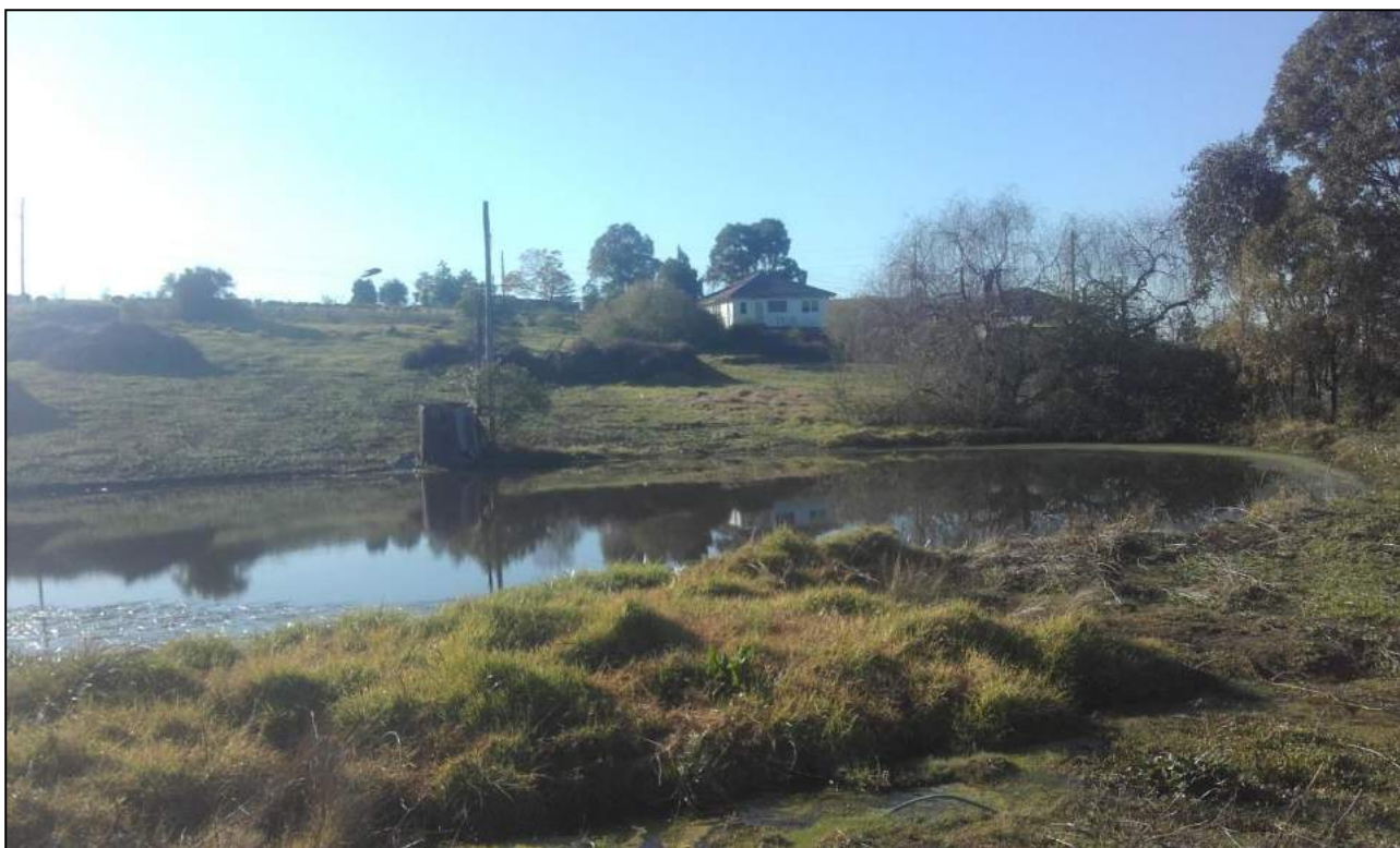
Photograph 7 – Northern section of Site, facing east across dam to property on Lot 18.
