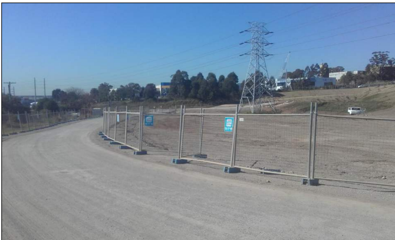
Photograph 17 – Southernmost section of Site, access road has been cut into Site for access to the construction site to the south.
