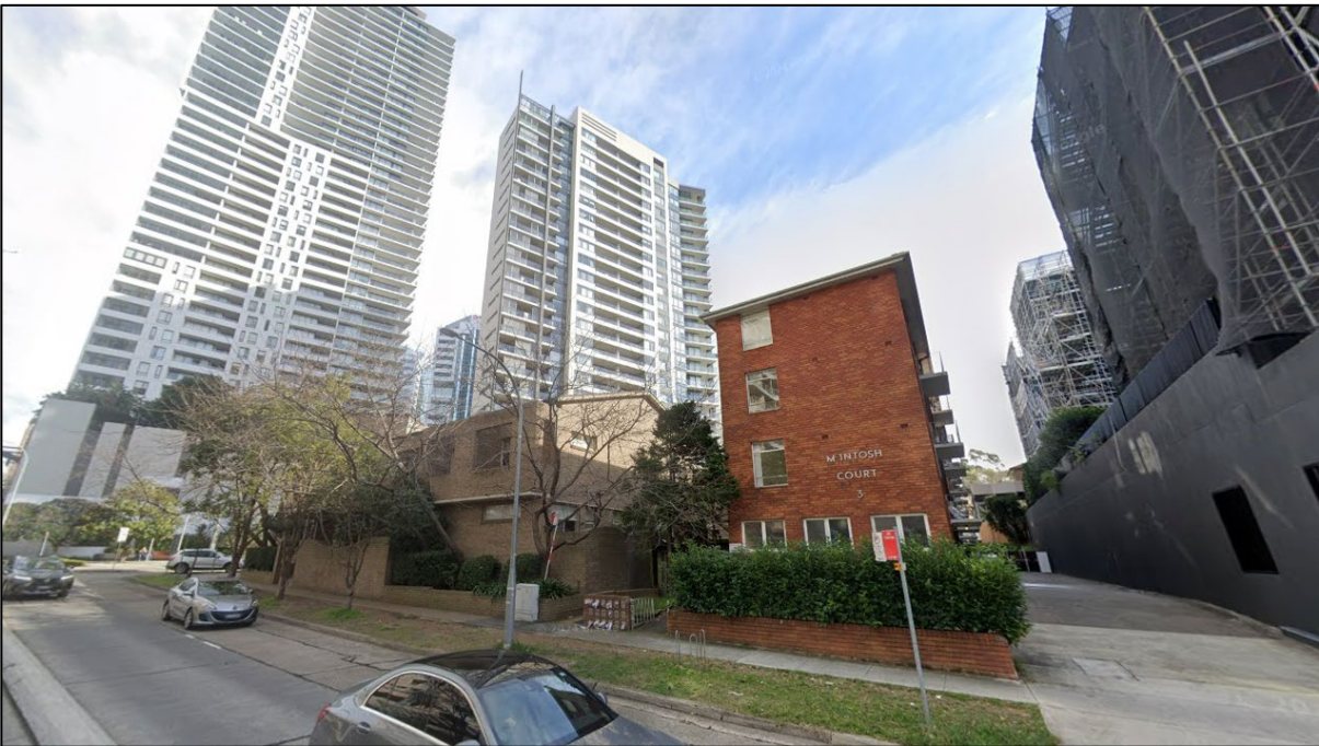
Figure 14: View of site from Help Street looking north-west Source: Google Streetview
