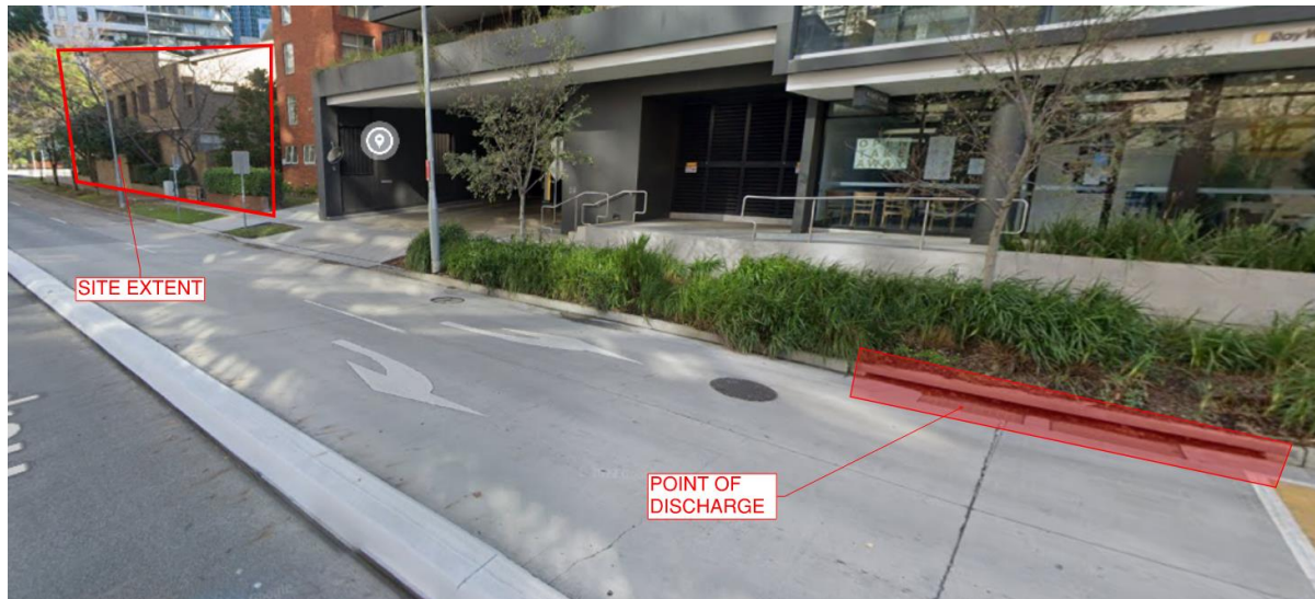
Figure 3: Site Image of Stormwater Infrastructure at Help Street
