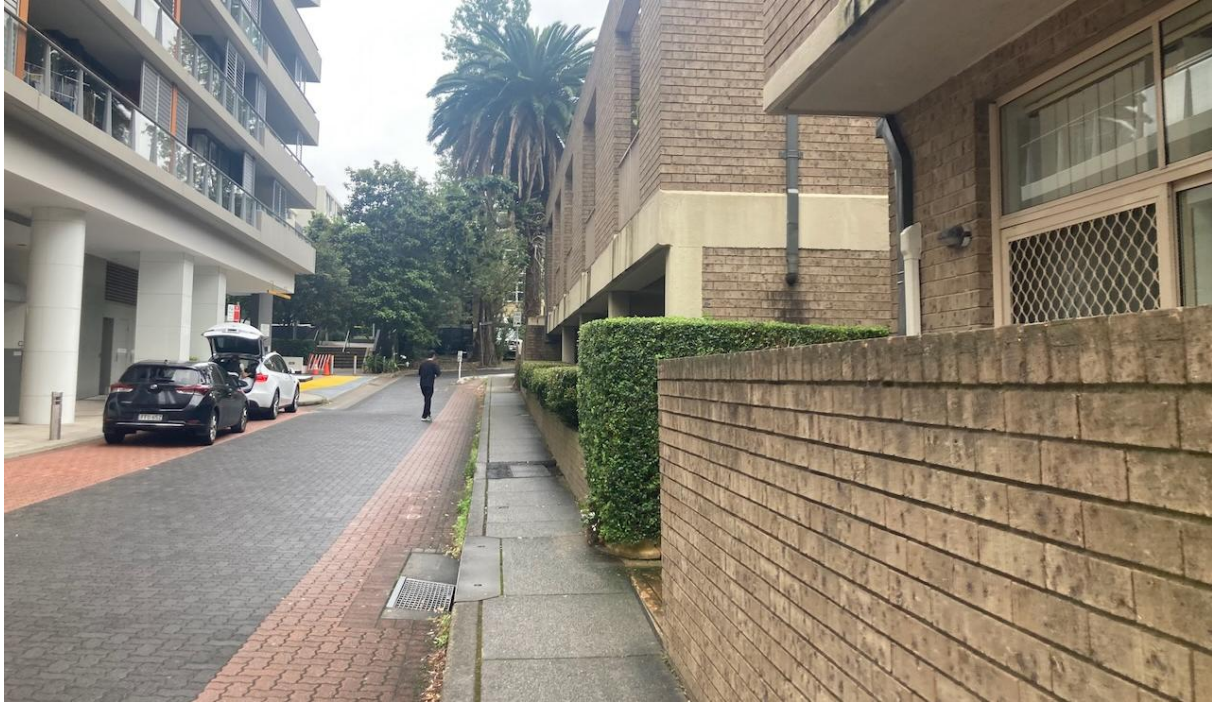
Figure 18: High brick walls of 5 Help Street, fronting Cambridge Lane
