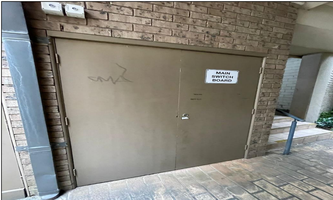
Photograph 20: 5 Help Street, main switch room, electrical cupboard, internal components, suspected asbestos.
