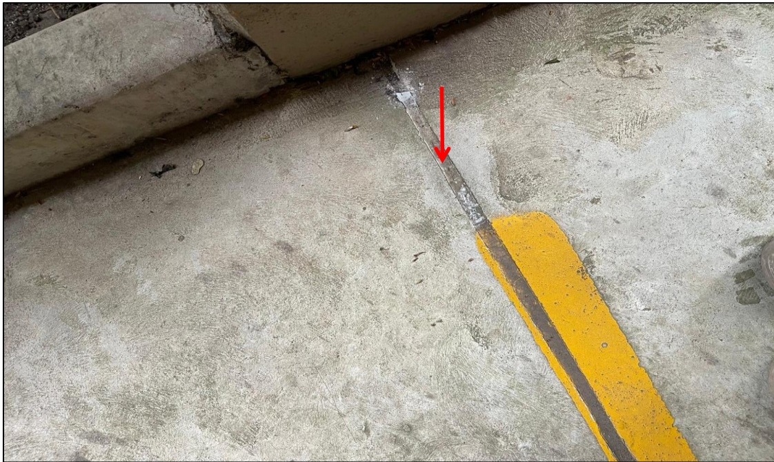
Photograph 12: 5 Help Street, exterior, car park area, joint in concrete, mastic, no asbestos detected by analysis.
