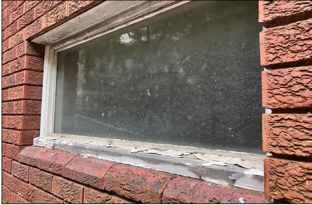
Photograph 17: 3 Help Street, exterior, typical window frame.
