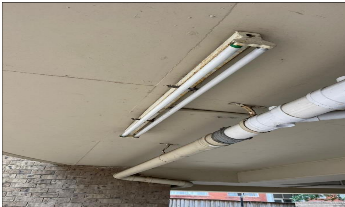
Photograph 24: 5 Help Street, exterior, car park area, ceiling, fluorescent light fittings, internal components (e.g., capacitors / ballasts), PCB (suspected).
