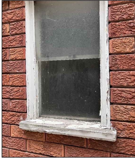
Photograph 19: 3 Help Street, exterior, eastern façade, southern end, window frame, white paint, lead paint detected.
