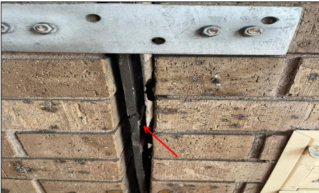
Photograph 14: 5 Help Street, exterior, southern entrance, wall, expansion gap, bituminous lining, no asbestos detected by analysis.
