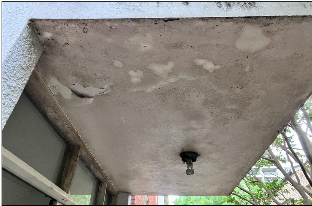
Photograph 18: 3 Help Street, exterior, western facade, northern end, concrete awning, white paint, may comprise lead paint.
