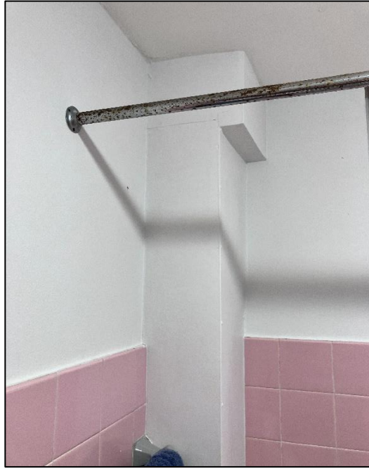
Photograph 27: 3 Help Street, Units 2, 7, 10 and 11, service conduits / risers, internal components, inaccessible.
