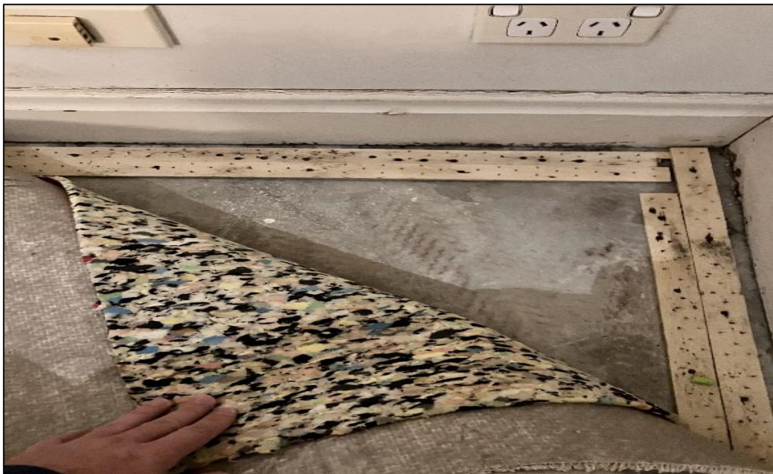
Photograph 4: 5 Help Street, Units 4, 11, 19 and 28, below floor coverings, substrate generally, suspected non-asbestos.
