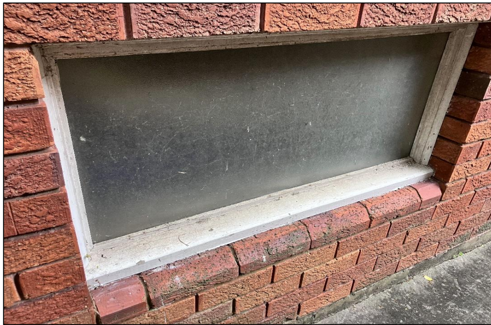
Photograph 16: 3 Help Street, exterior, typical window frame.
