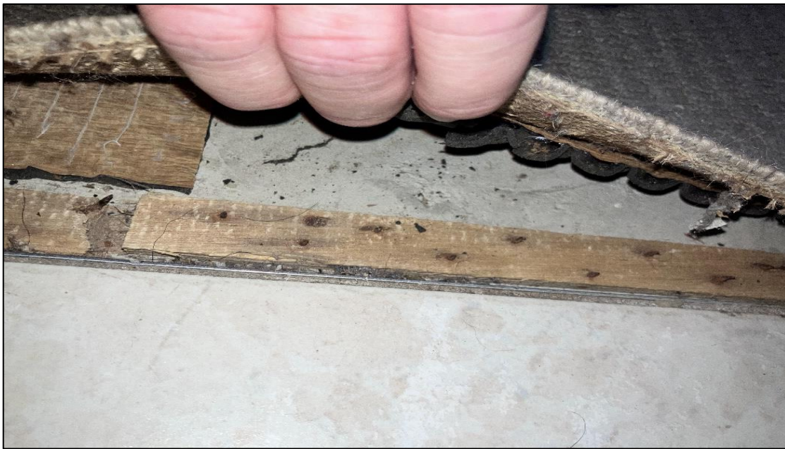
Photograph 5: 5 Help Street, Units 4, 11, 19 and 28, below floor coverings, substrate generally, suspected non-asbestos.
