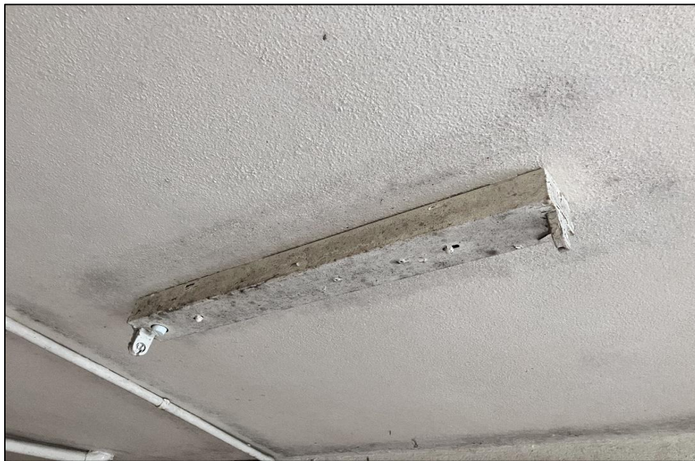
Photograph 24: 3 Help Street, ground floor, Laundry, fluorescent light fittings, internal components (e.g., capacitors), PCB (suspected).
