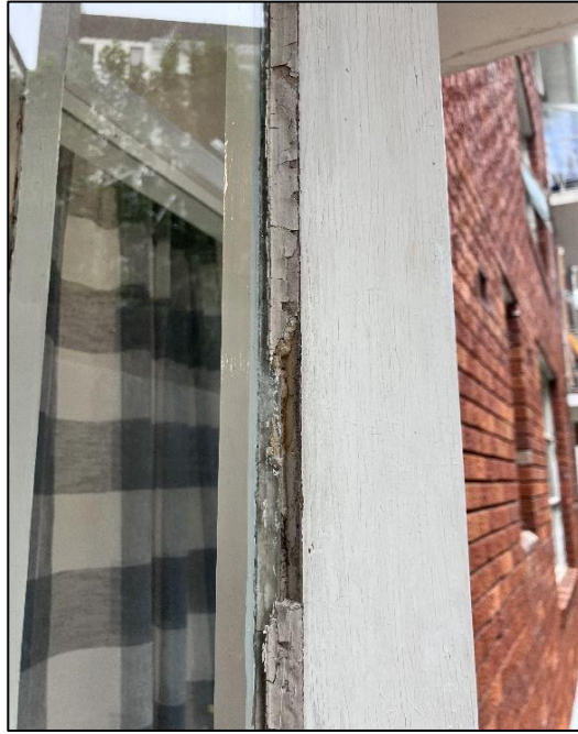
Photograph 29: 3 Help Street, typical balcony, door, glazing putty, no asbestos detected by analysis.
