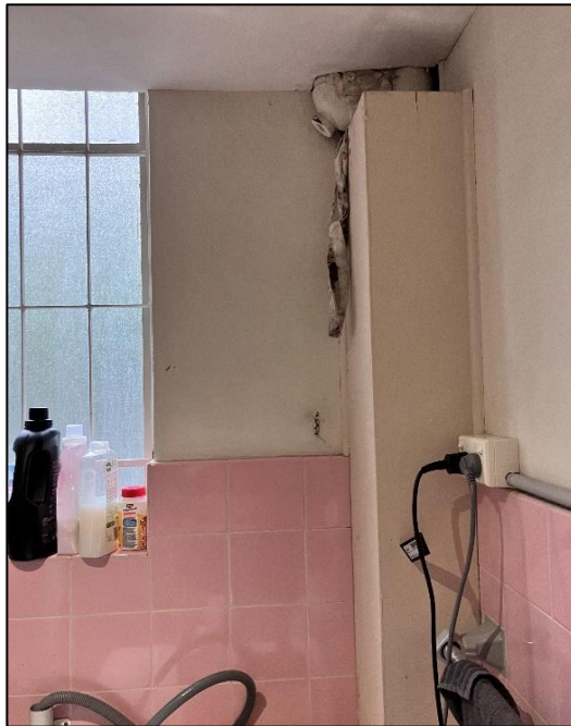
Photograph 28: 3 Help Street, Units 2, 7, 10 and 11, service conduits / risers, internal components, inaccessible.
