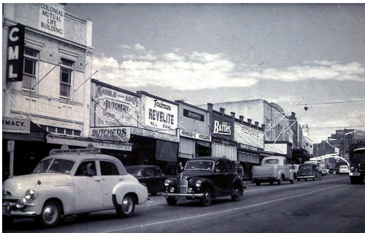
Figure 3.14 c.1950 – 1960 photograph Crown Street shops.
