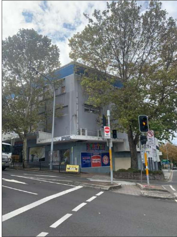
Figure 16: South western corner. This section lies under the roof form marked '3' in Figure 4.
