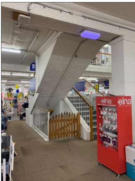
Figure 23: Detail of the pressed metal beneath the staircases and the pressed metal cornice to beams. WP Heritage, 2021.
