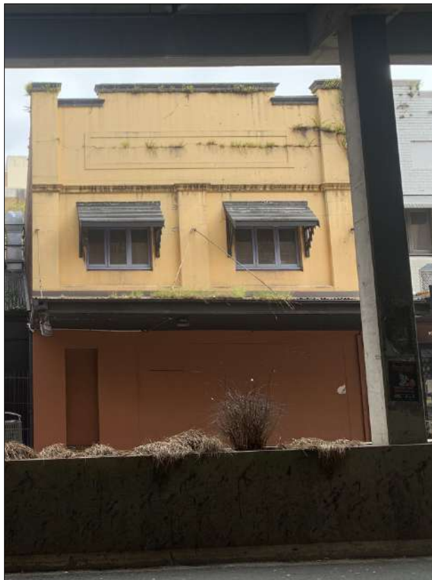
Figure 33: No. 232-234 Keira Street.
