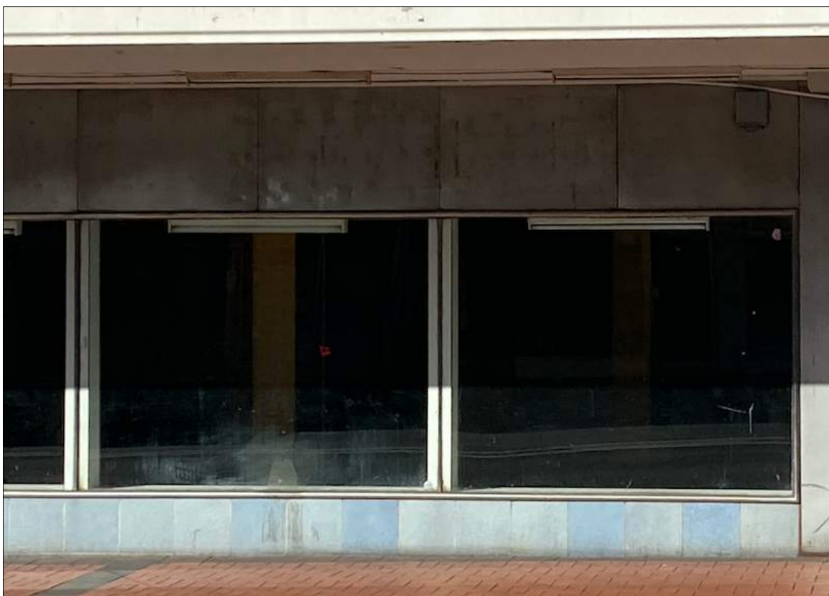
Fig. 14. Curved stainless steel frame to glass shopfronts and signage is to be retained and protected from damage during all approved building works.
