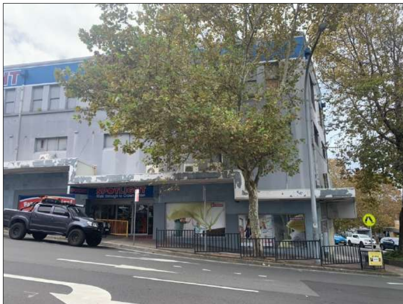
Figure 14: Continuing south along the western elevation. This section lies under the roof form marked '3' in Figure 4.
