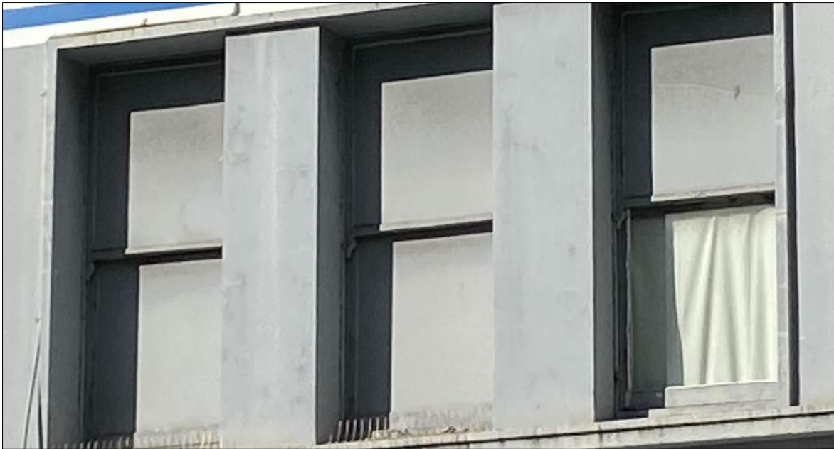
Fig. 27. All the double hung timber windows in the façade in both Atchison and Crown Street are to be restored.
