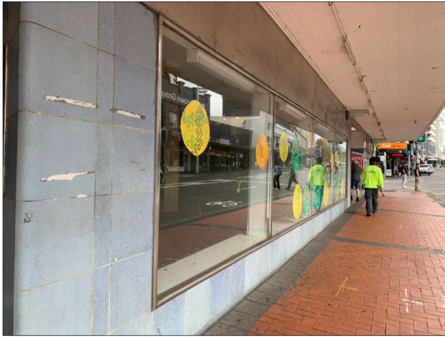
Figure 8: Looking along the Crown Street elevation, showing the large metal framed shop windows.
