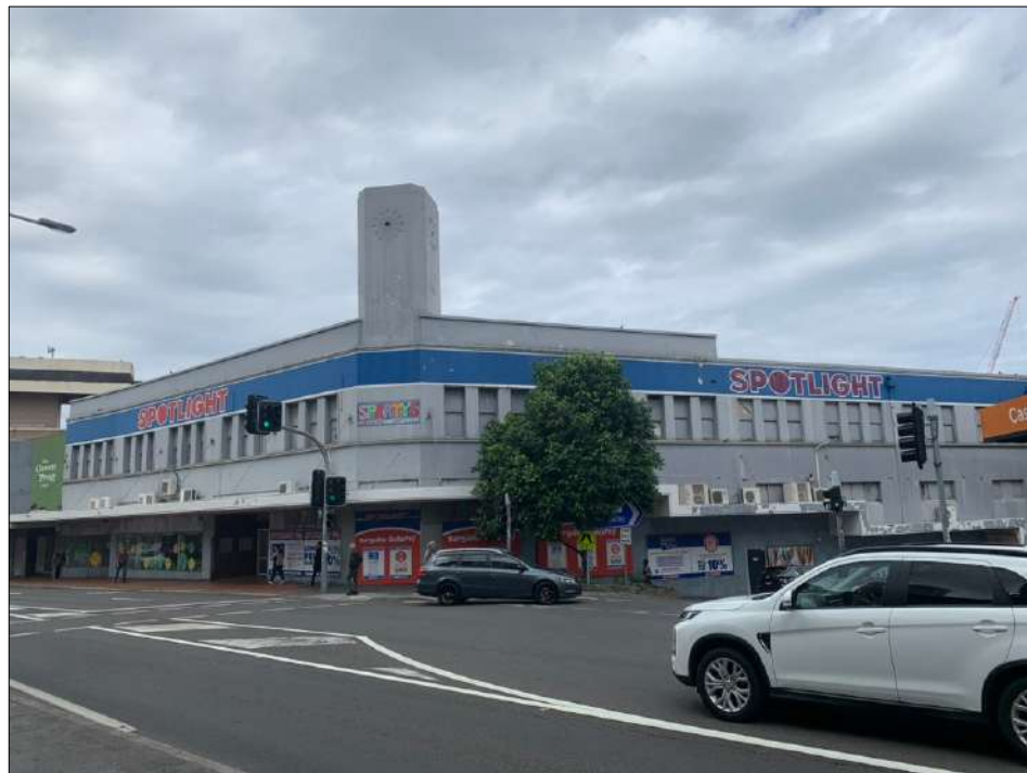
Figure 7: The north western corner of the building.
