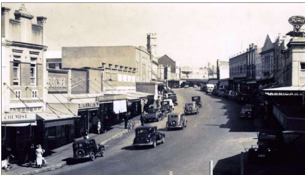
Figure 60: Crown Street, 1945. Showing the building in its setting. This photograph also shows the other buildings, since demolished or substantially altered, on the larger site of the proposed development.
