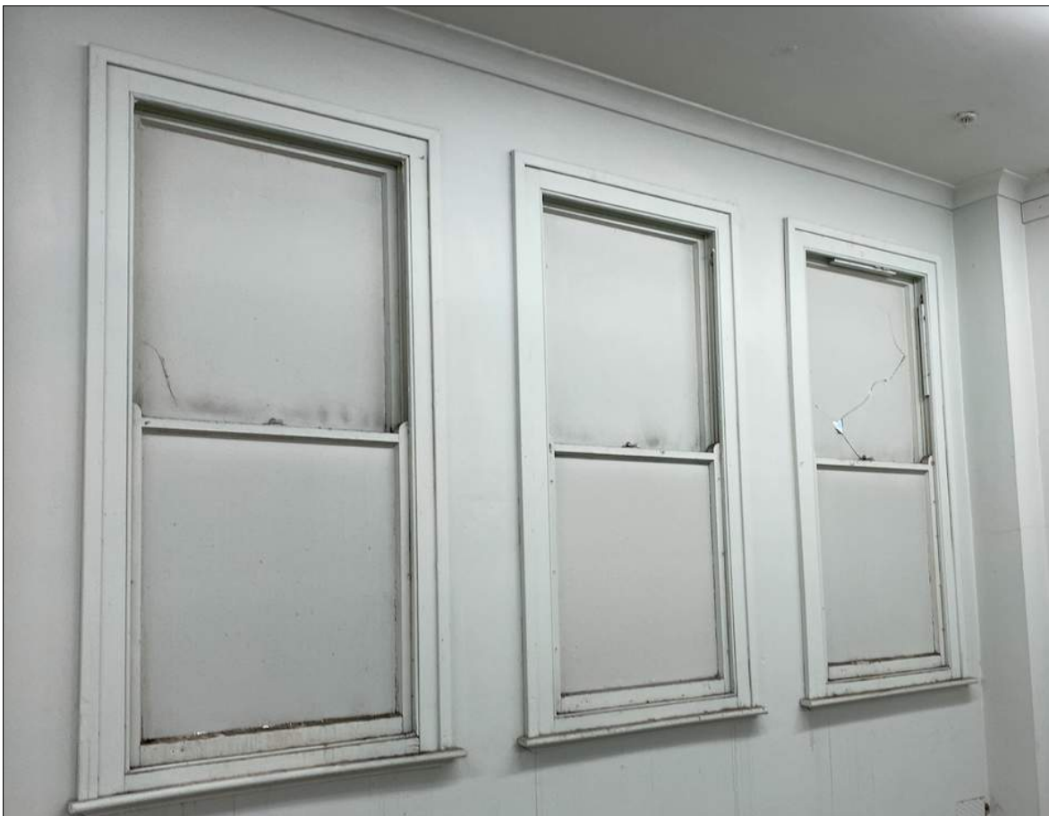
Fig. 30. All the double hung timber windows in the façade in both Atchison and Crown Street are to be restored.
