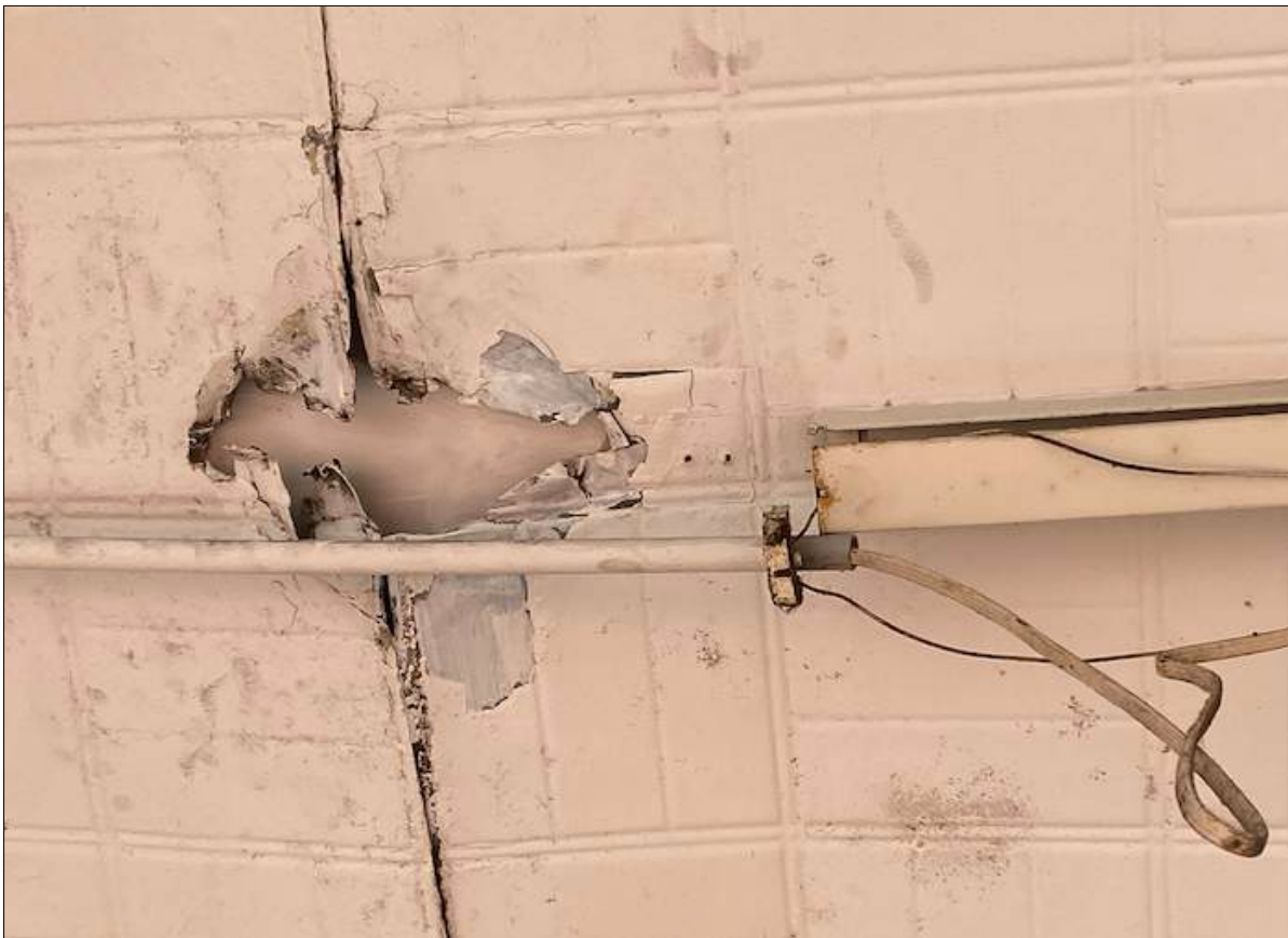
Fig. 41. Awning soffits (pressed metal ceilings) are to be retained, repaired prior to proper preparation and repainting.
