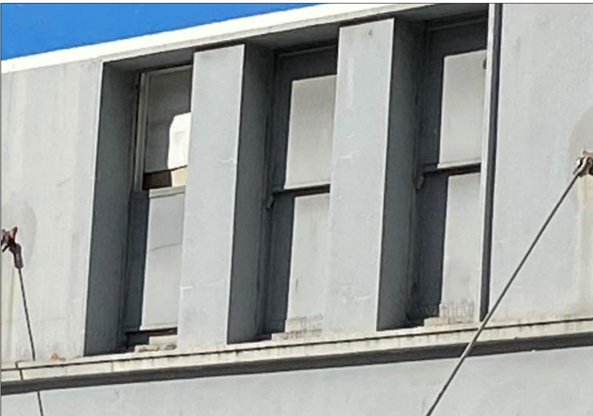
Fig. 26. All the double hung timber windows in the façade in both Atchison and Crown Street are to be restored.
