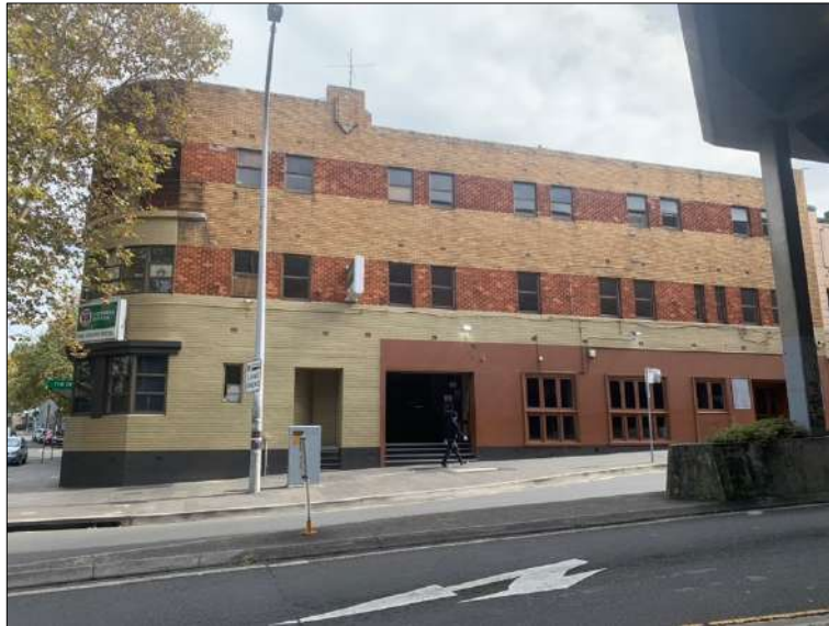
Figure 35: Kiera Street elevation of the Grand Hotel.
