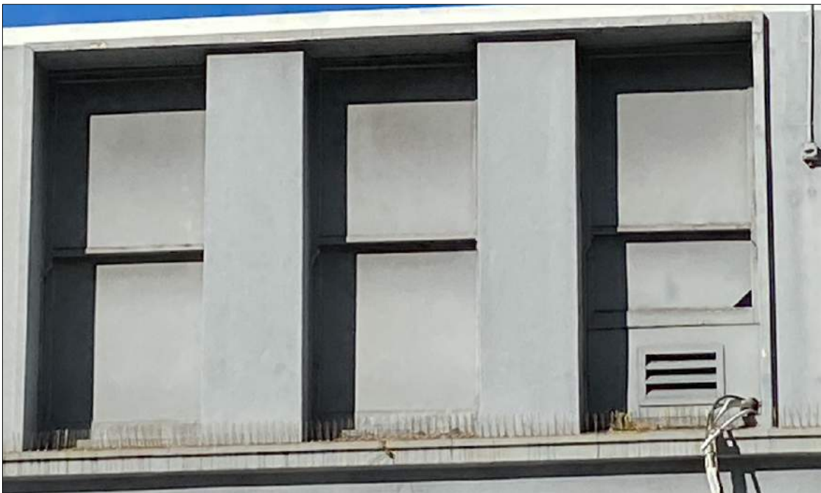
Fig. 28. All the double hung timber windows in the façade in both Atchison and Crown Street are to be restored.
