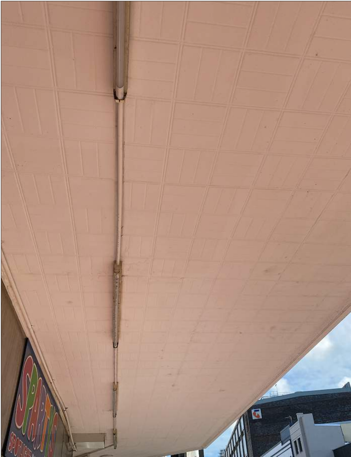
Fig. 39. Awning soffits (pressed metal ceilings) are to be retained, repaired prior to proper preparation and repainting.
