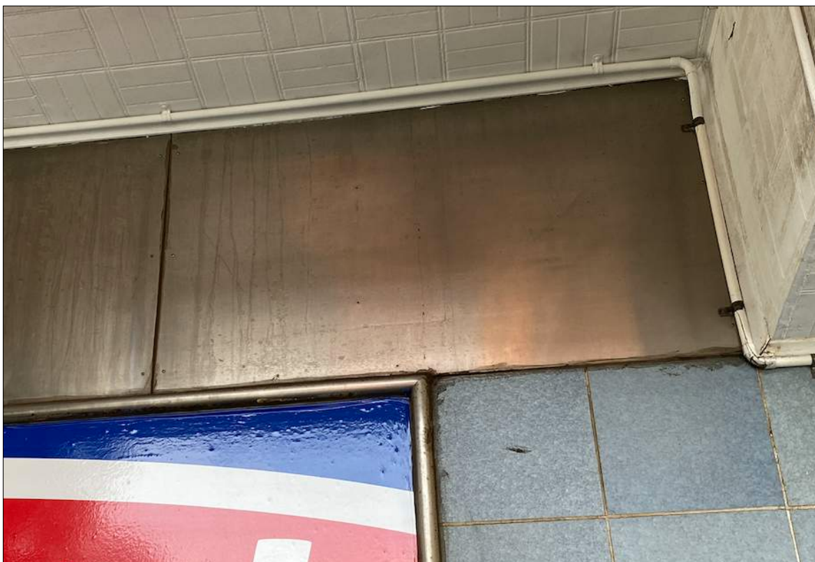
Fig. 13. Curved stainless steel frame to glass shopfronts and signage is to be retained and protected from damage during all approved building works.
