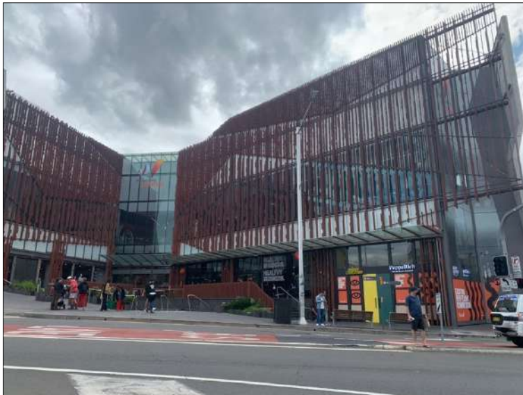
Figure 46: Glass and steel building on the corner of Crown Street and Kiera Street, opposite the site.
