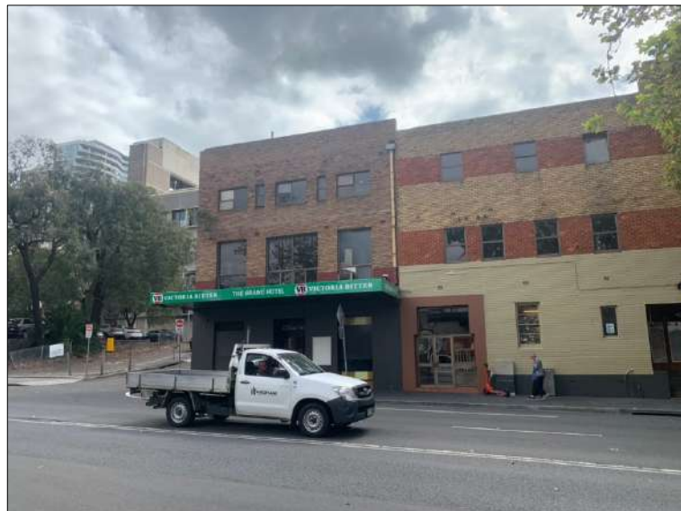
Figure 38: Western end of the Burelli Street elevation, showing the 1956 addition.
