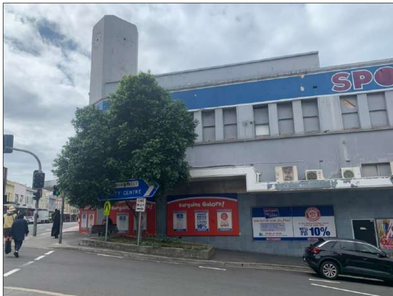
Figure 12: Western elevation. This section lies under the roof forms marked '2' and '3' in Figure 4.
