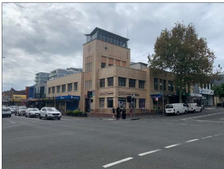
Figure 83: National Mutual Life Assurance Building, Keira Street.
