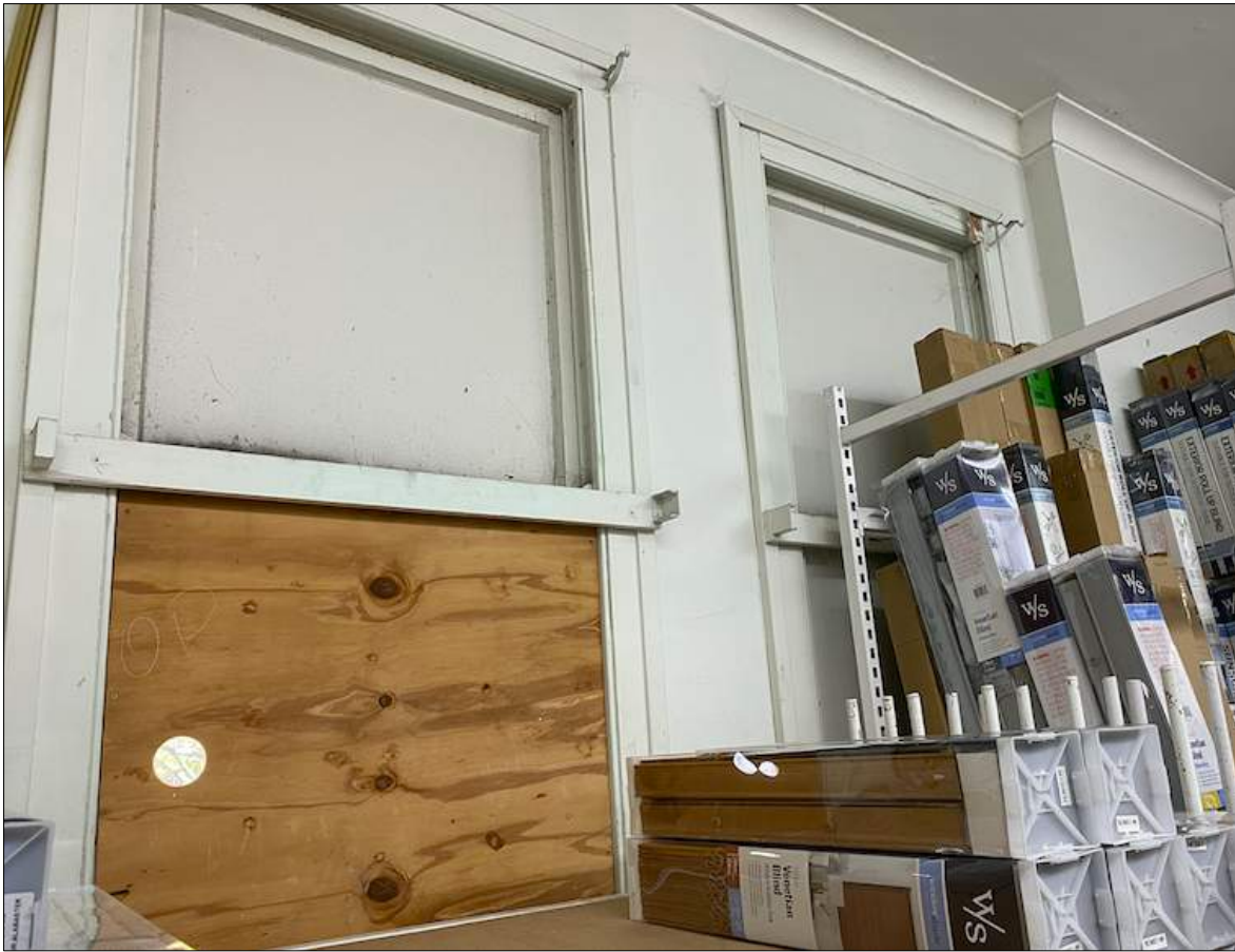
Fig. 31. All the double hung timber windows in the façade in both Atchison and Crown Street are to be restored.
