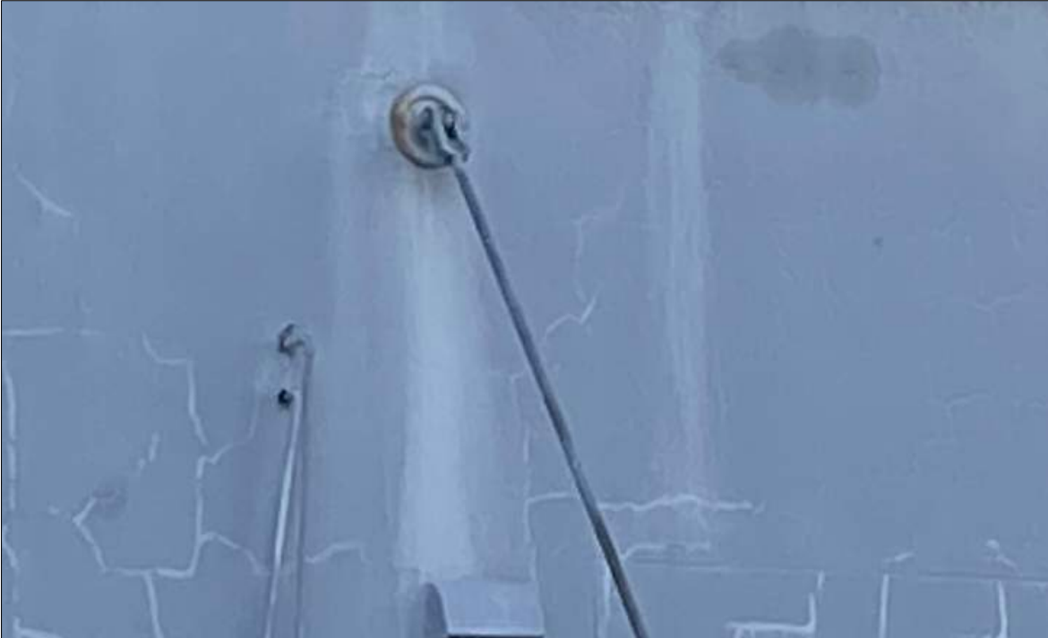
Fig. 37. All Support suspension anchors and suspension elements are to be properly inspected by an experienced awning installation contractor with a history of satisfactory work on heritage buildings.
