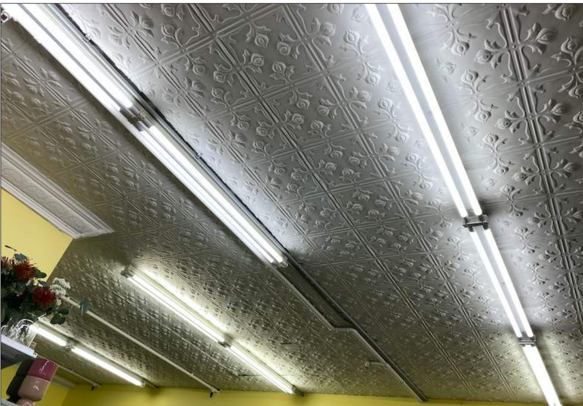
Fig. 43. The pressed metal ceilings of the lower ground floor are to be salvaged where ever possible, protected from damaged and recycled either in the new construction in a nominated area and/or offered to a heritage building centre.
