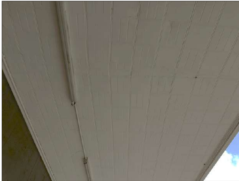
Figure 11: Detail of the asbestos tile sheeting to the underside of the awning.
