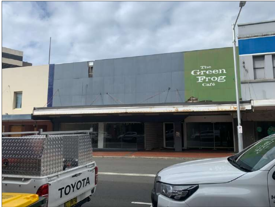
Figure 5: Eastern most end of the building on the heritage listed site, Crown Street elevation.
