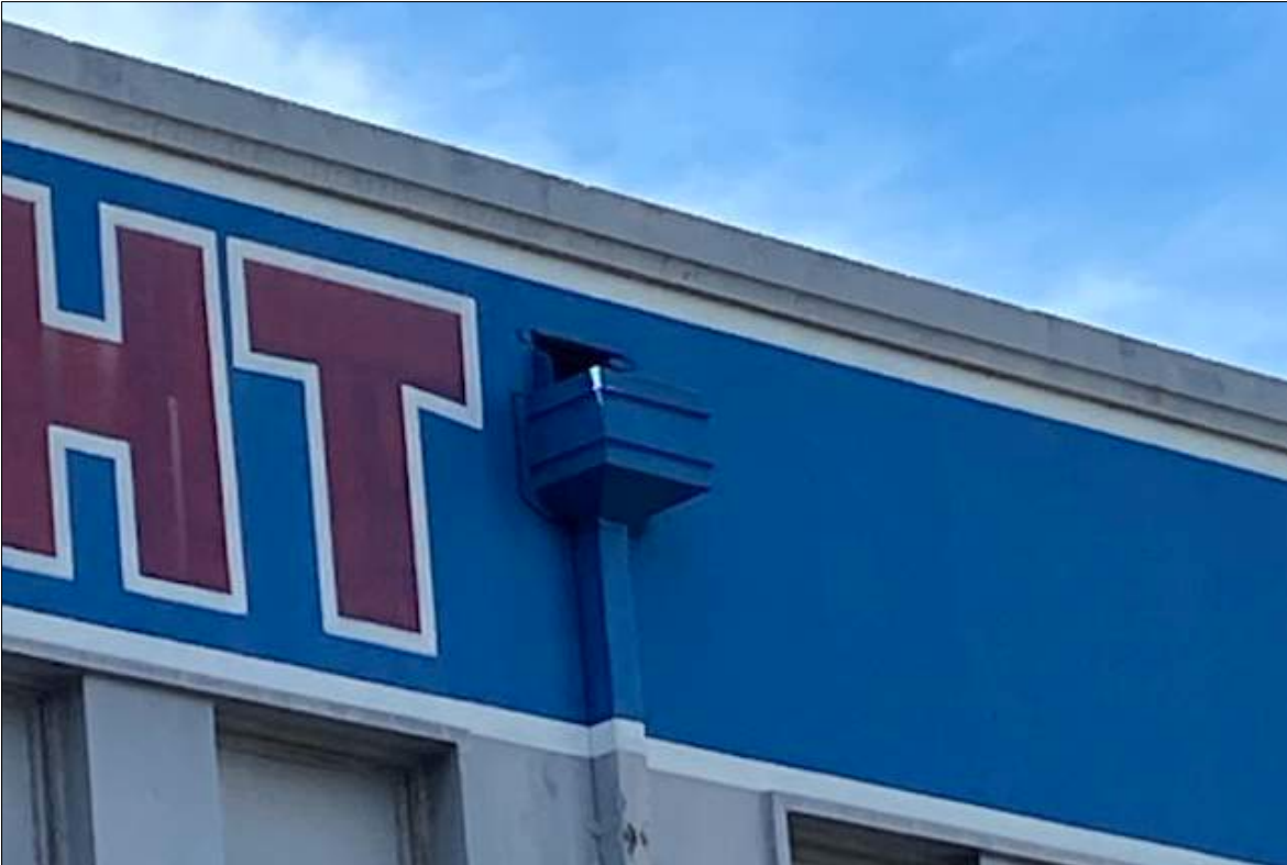
Fig. 25. The rain-heads and down-pipes on the Atchison Street façade are to be retained or replaced with 'like-for-like' rain-heads and down-pipes if corroded beyond repair.
