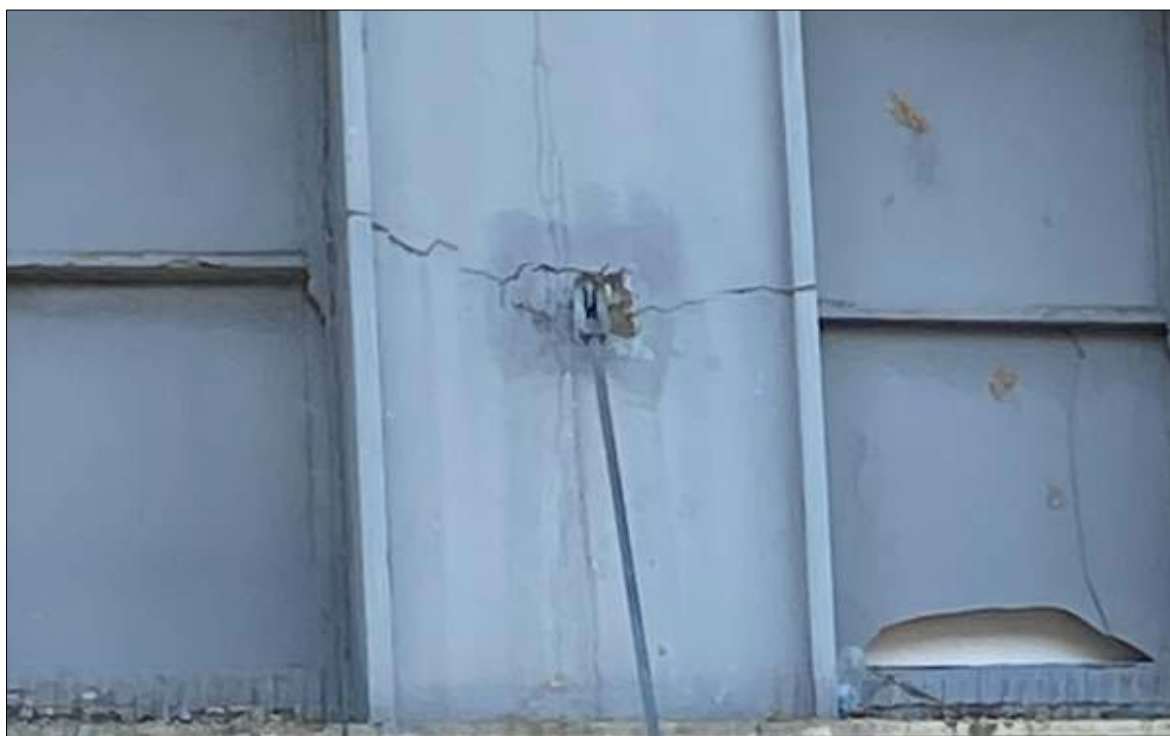
Fig. 36. All Support suspension anchors and suspension elements are to be properly inspected by an experienced awning installation contractor with a history of satisfactory work on heritage buildings.
