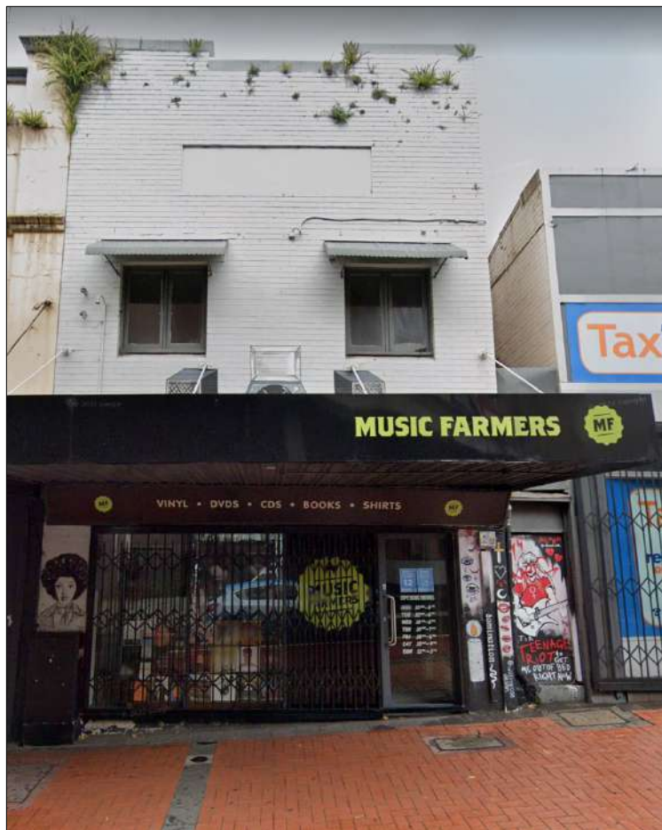
Figure 32: No. 226-230 Keira Street.
