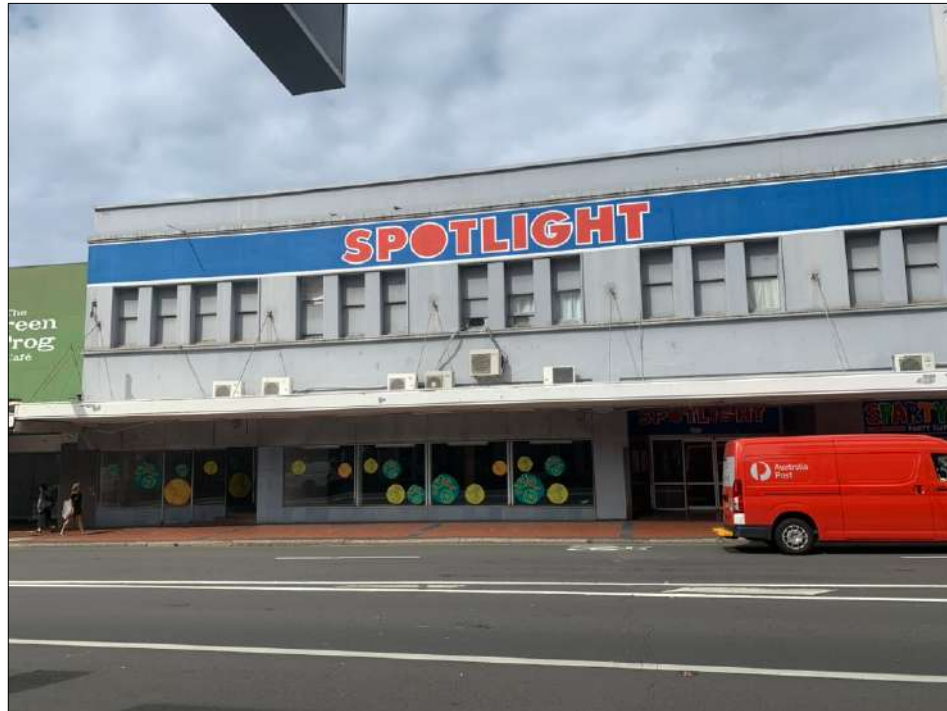
Figure 6: Northern elevation of the western building.
