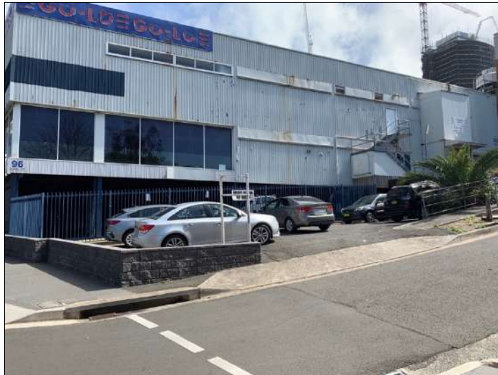
Figure 20: Eastern elevation of the later addition.
