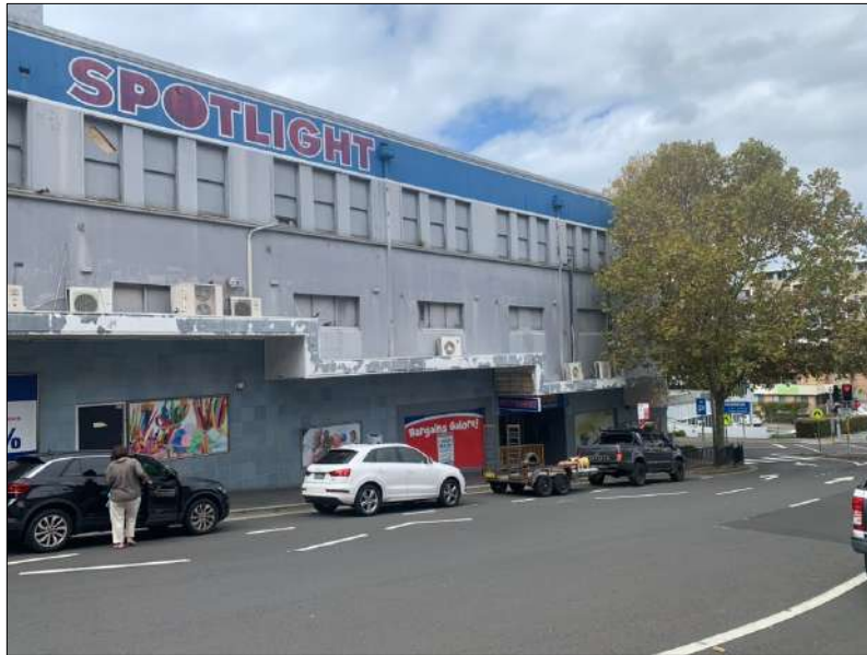
Figure 13: Continuing south along the western elevation. This section lies under the roof form marked '3' in Figure 4.
