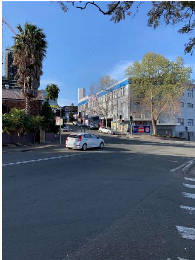
Figure 81: View towards the site on approach along Burelli Street from the south west. The western elevation and the clock tower are now visible. WP Heritage and Planning 2021.
