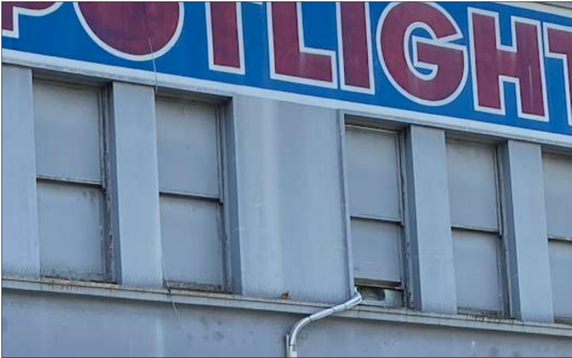
Fig. 29. All the double hung timber windows in the façade in both Atchison and Crown Street are to be restored.
