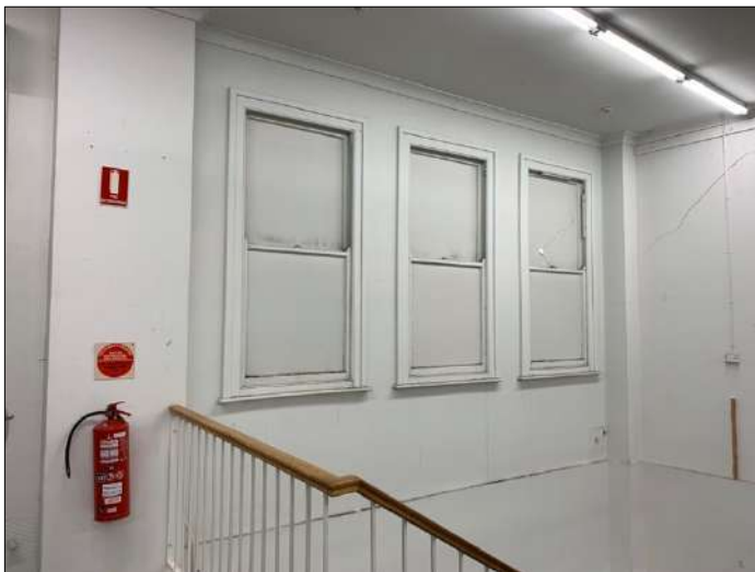
Figure 30: Typical window joinery at first floor level. WP Heritage, 2021.
