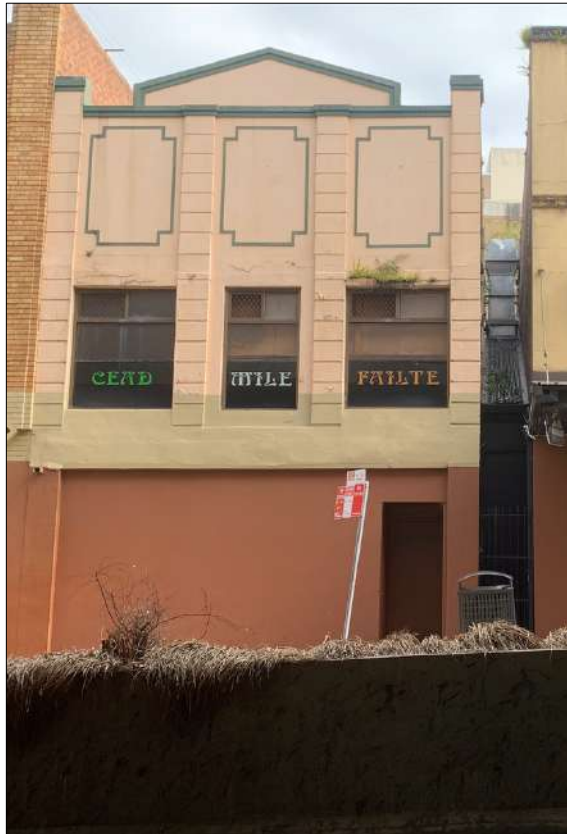
Figure 34: No. 236-238 Keira Street.
