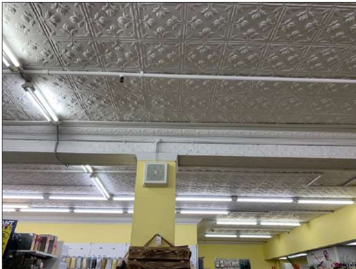
Figure 22: Detail of the pressed metal ceiling at basement level. WP Heritage, 2021.
