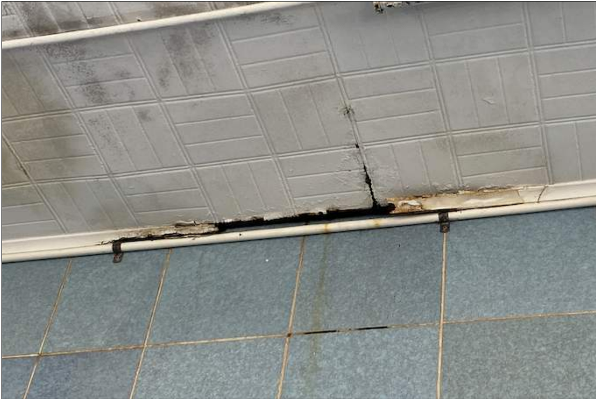
Fig. 40. Awning soffits (pressed metal ceilings) are to be retained, repaired prior to proper preparation and repainting.
