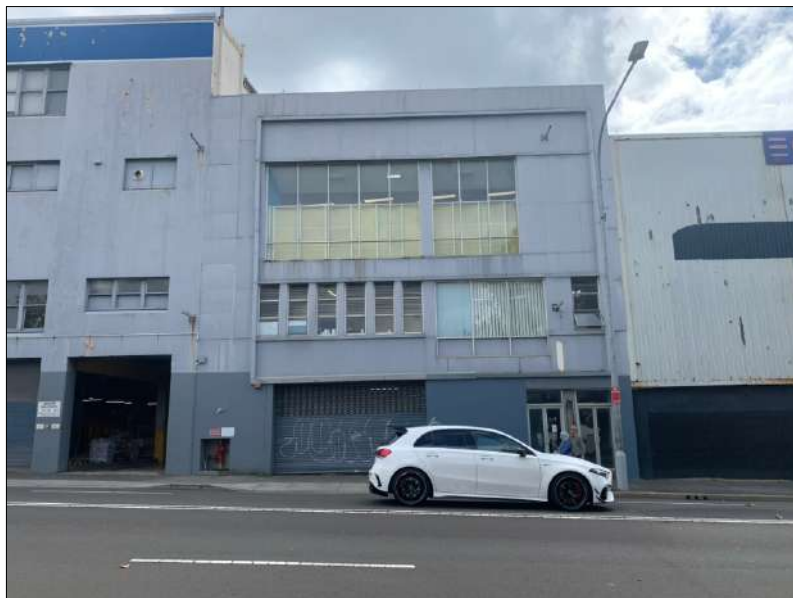
Figure 18: Eastern end of the southern elevation.
