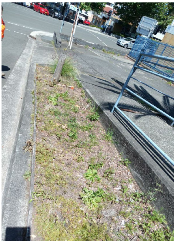
Figure 24: Soil exposure within the southern carpark. View south
