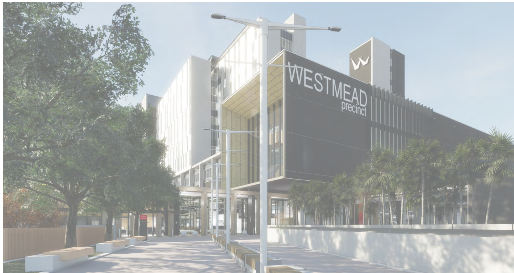
View of new CASB and Innovation Centre from Plaza
