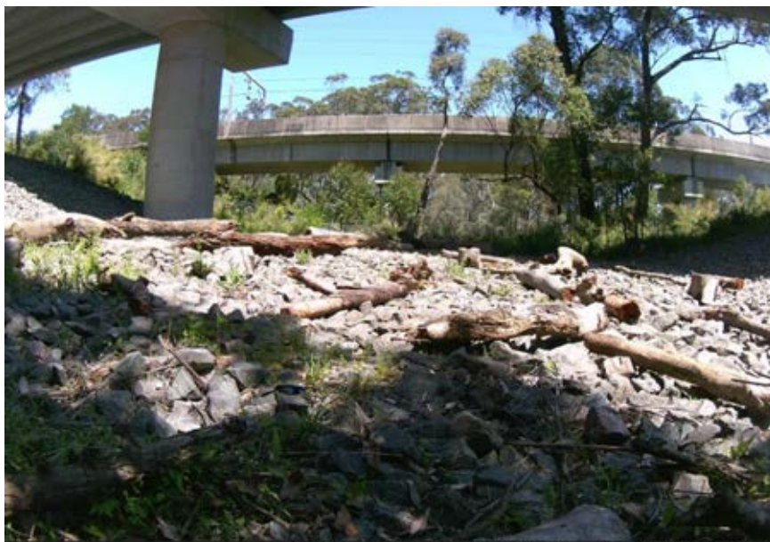
Plate 4-1. Large logs and piles of coarse woody debris placed to facilitate movement of fauna across ballast at Georges River beneath the rail link bridge
