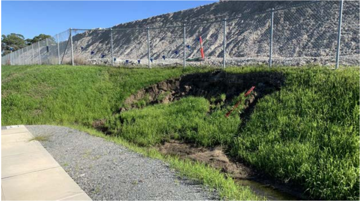
Plate 4. A section of soft batter within the Rail Link which has slipped following periods of high rainfall
