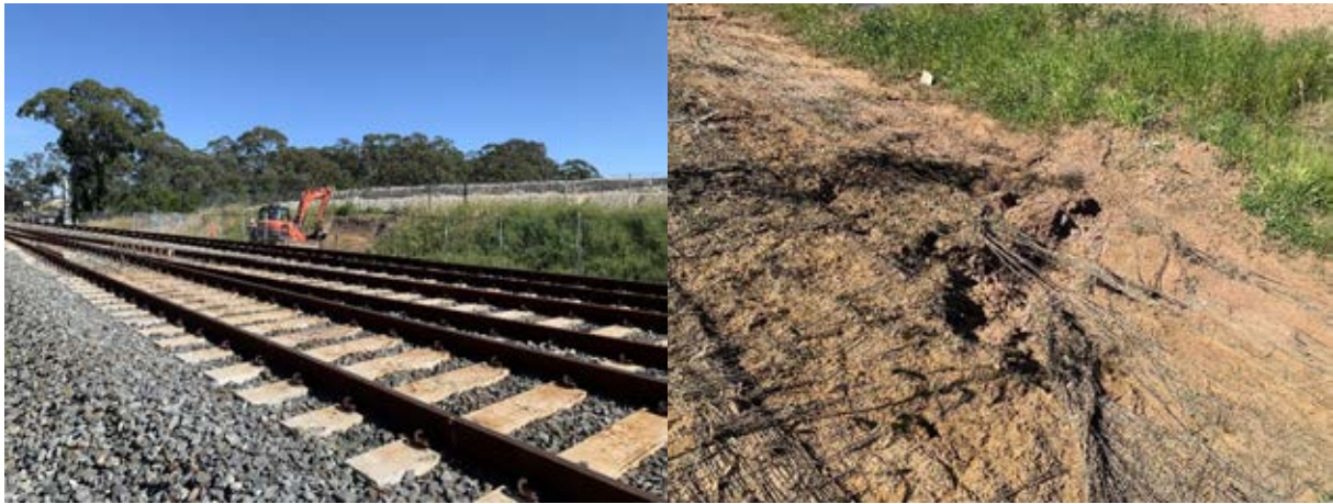
Plate 5. A section of soft batter within the Rail Link being remediated following a slip, and a new instance of batter slip within the MPE operational area
