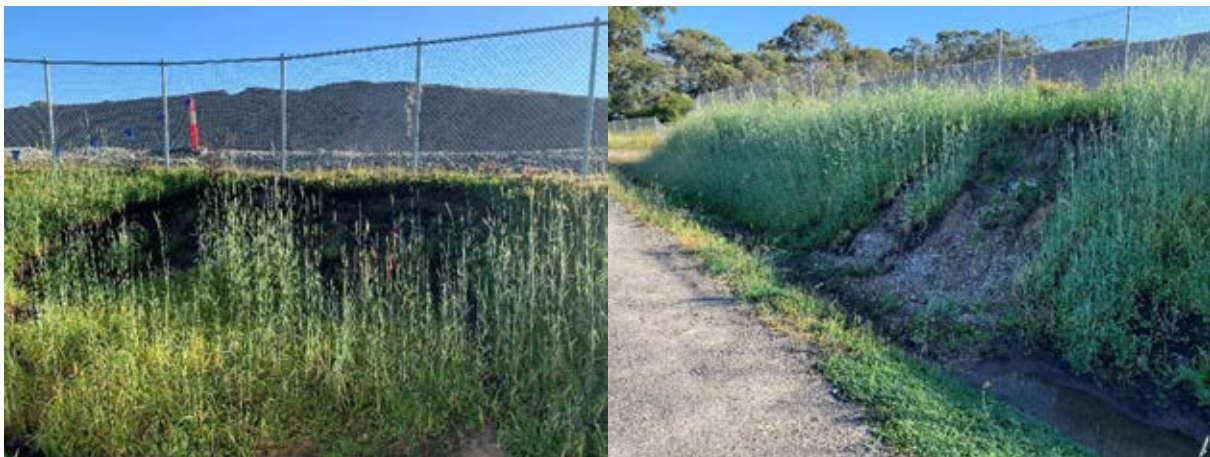
Plate 6. Two sections of soft batter within the Rail Link which have slipped following periods of high rainfall
