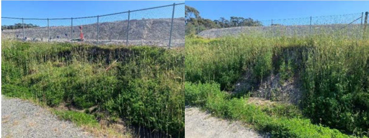
Plate 5. Two sections of soft batter within the Rail Link which have slipped following periods of high rainfall
