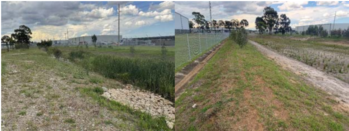
Plate 1. Low levels of weeds and established native plants observed on soft batters surrounding the basins and drainage channel at the north-eastern extent of the operation facility
