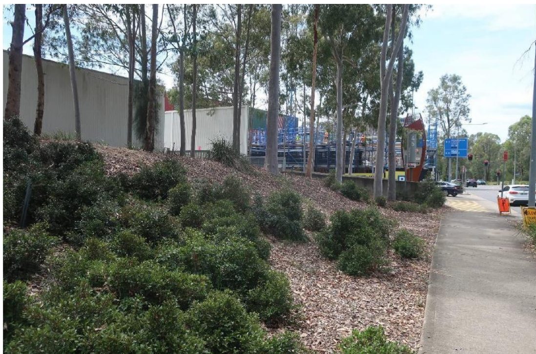
Figure 4-2 Study site facing north, showing built up earth mound. AMAC Group, 14/10/2024, IMG_8768.
