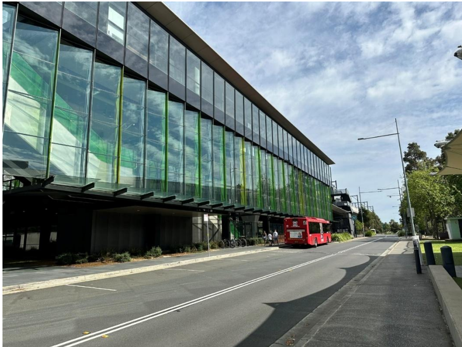
Figure 11: Rouse Hill Metro Station (Source: Keylan)
