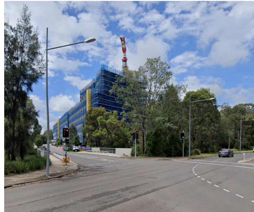
Figure 10: View looking south of White Hart Drive (Source: Google Maps)
