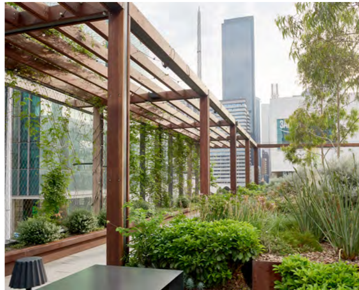
SHADE STRUCTURE ROOFTOP
