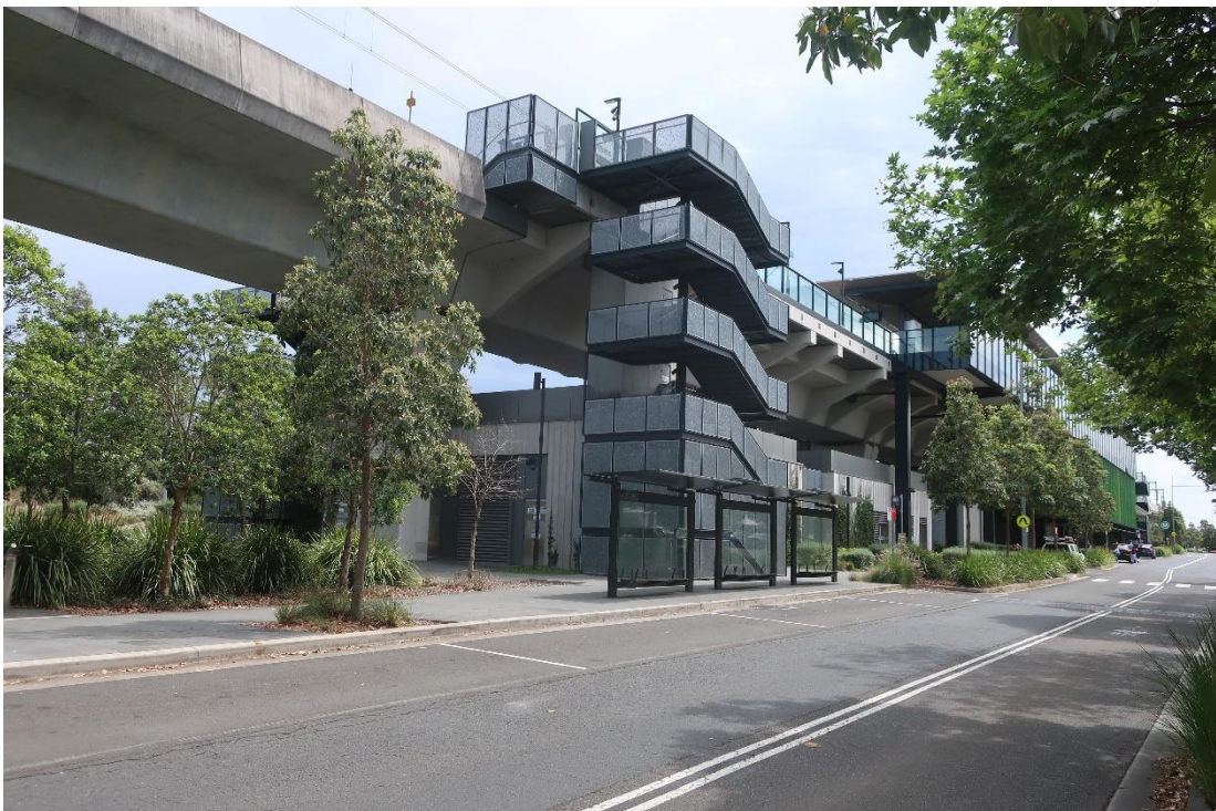
Figure 1.15 View from southern site boundary looking towards Rouse Hill metro station. Facing southwest. AMAC Group, 14/10/2024, digital image 8753.
