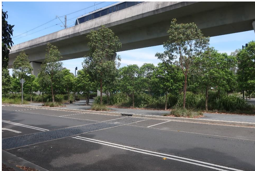
Figure 4.1 Windsor Road alignment concealed from Tempus Street ground level. Facing southeast.
