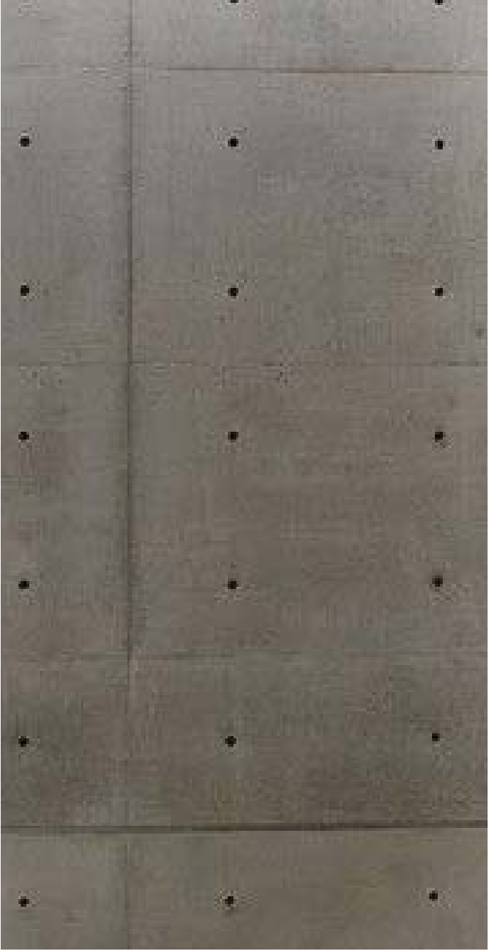
CO - 1 EXAMPLE OF OFF FORM CONCRETE TADAO ANDO
