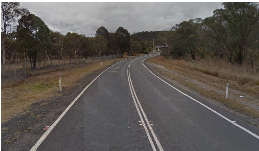
Figure 2 Castlereagh Highway viewed northwards towards Boulder Road
