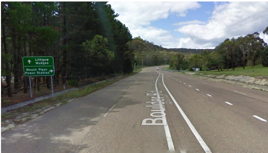
Figure 3 Boulder Road viewed northwards towards Castlereagh Highway
