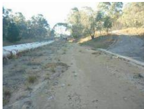
Plate 33 Existing pipeline Skelly Rd view north
