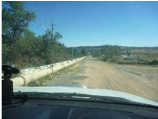
Plate 34 West of LDP009 pipeline & access road
