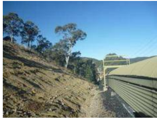
Plate 31 Conveyor near Wolgan & Skelly Roads
