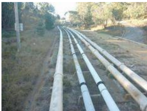
Plate 32 Existing pipeline Skelly Rd view north
