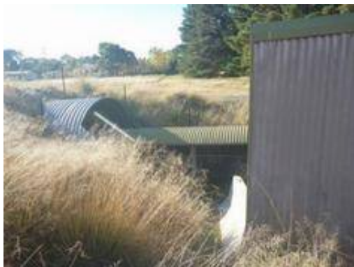
Plate 28 Conveyor Tunnel – view north
