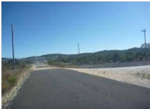
Plate 3 Formed roads in MPPS - view to west
