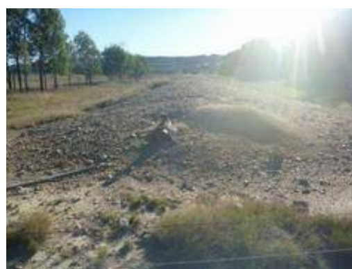
Plate 27 View west along top of conveyor tunnel
