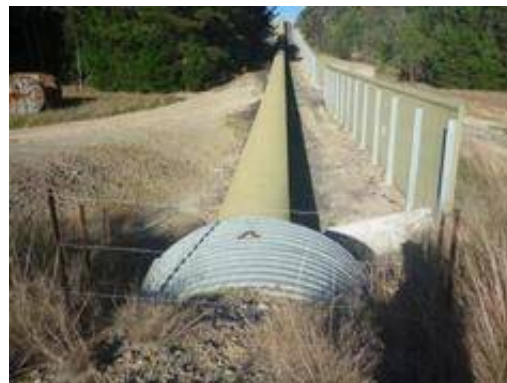
Plate 29 Conveyor area - view east
