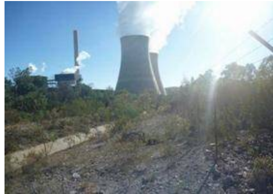
Plate 2 View north west showing culvert
