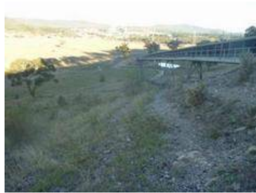
Plate 25 View north east from conveyor
