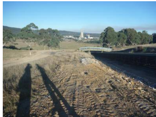
Plate 23 Overland conveyor area view east
