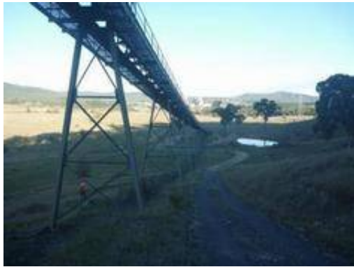
Plate 24 Modified land surface near conveyor
