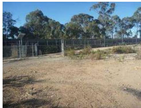
Plate 16 View south -clearing mid slope area
