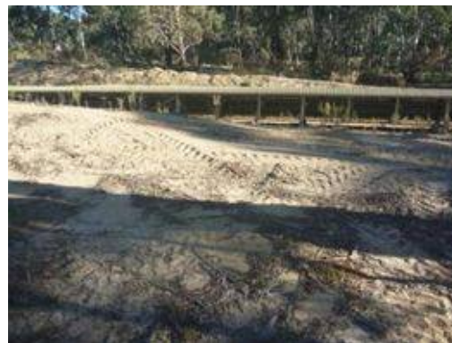
Plate 18 Conveyor area view south
