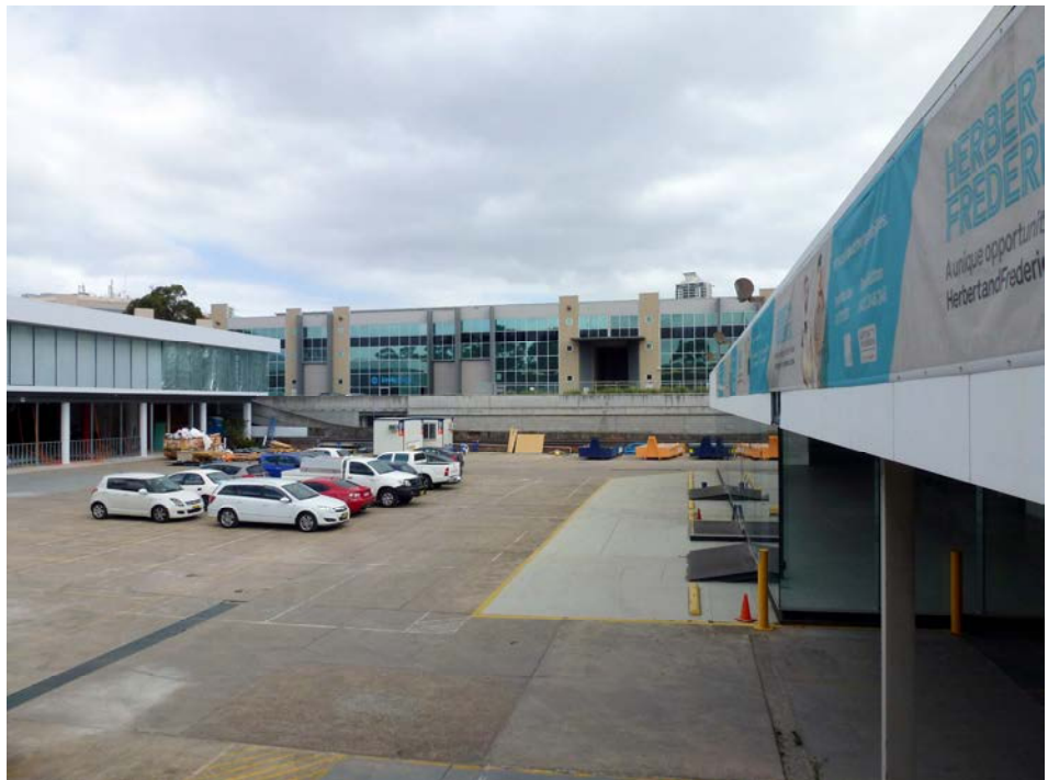
Figure 3 – Existing hardstand and Building (right)
