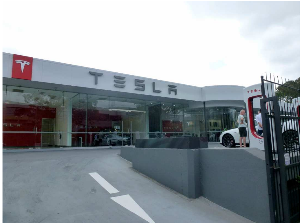
Figure 4 – Car showroom to the north east of the site
