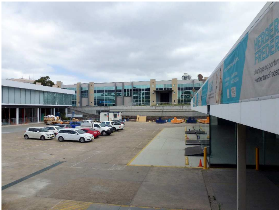
Figure 8 – Existing hardstand and building (right)
