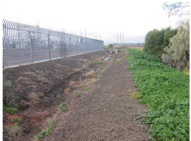
Plate 6.8 View north along the perimeter of the Narrabri Substation, showing a graded easement and shallow drainage channel adjacent to the secure compound.
