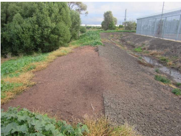
Plate 6.7 Heavily modified ground surface adjacent to the Narrabri Substation, showing compacted reddish-brown fill material and imported gravel, view north
