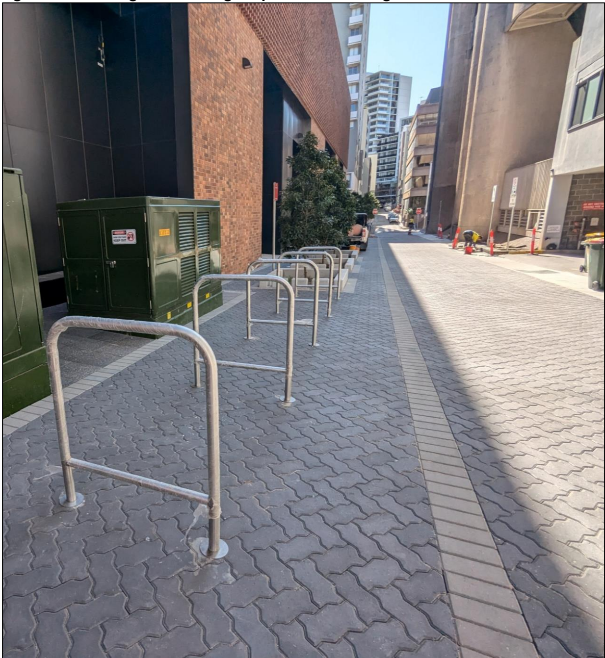
Figure 2.8: Existing Surrounding Bicycle Racks along Clarke Lane
