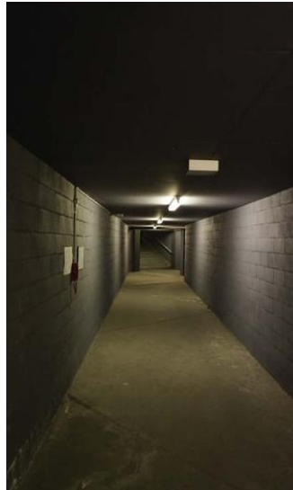
Existing fire tunnel
