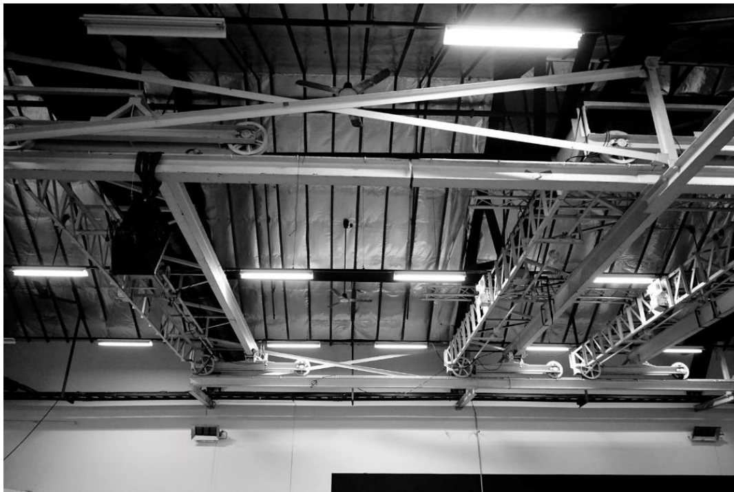
Figure 40: Gantry cranes at Level 1. Photo by Hassell.
