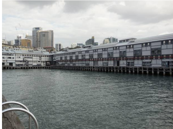
Figure 6: Wharf 4/5 East elevation
