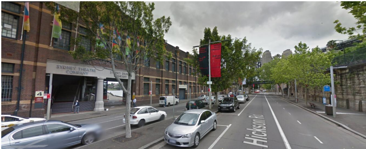
Figure 15: Hickson Road looking North/East. Image by Google.
