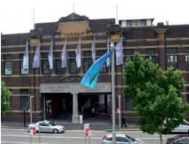
Figure 11: Shore Sheds South elevation
