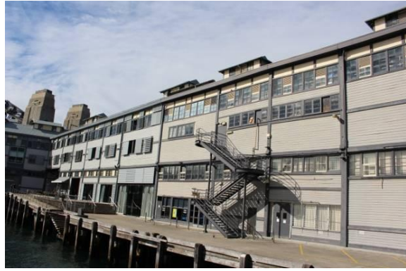
Figure 14: Fire escapes in steel
