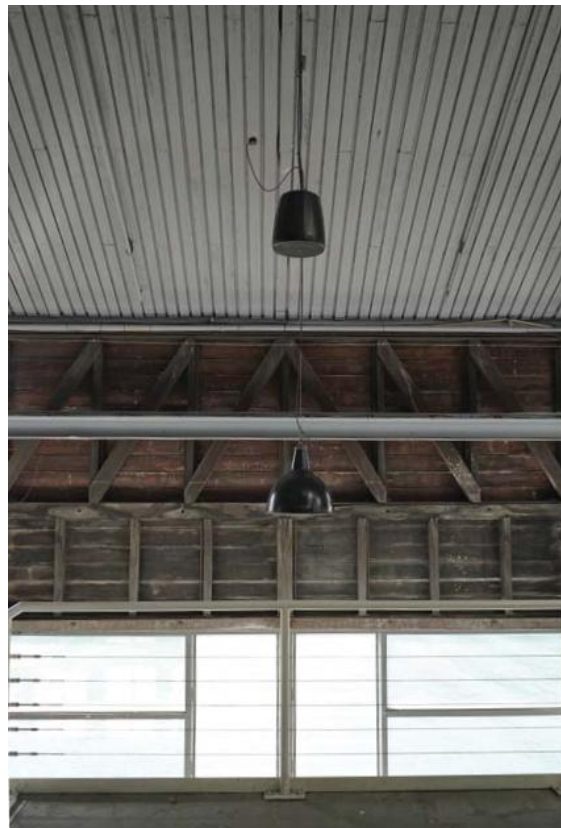
Figure 35: Existing timber batten ceiling
