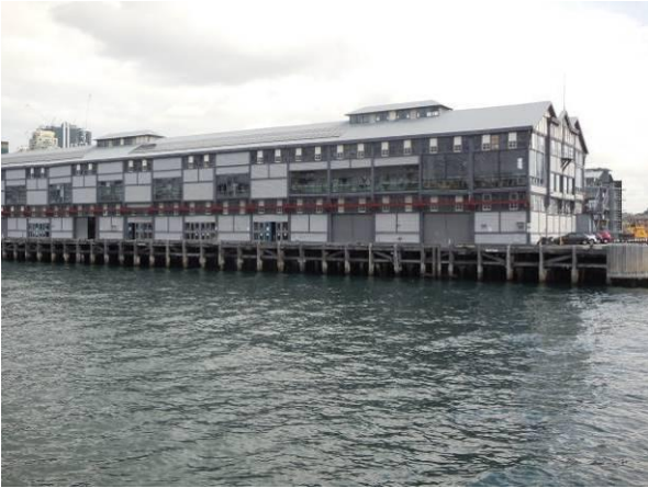
Figure 5: Wharf 4/5 East elevation
