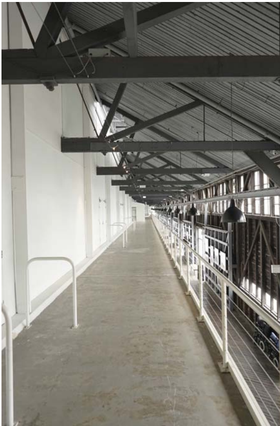
Mezzanine Level / Fire Tunnel Under
