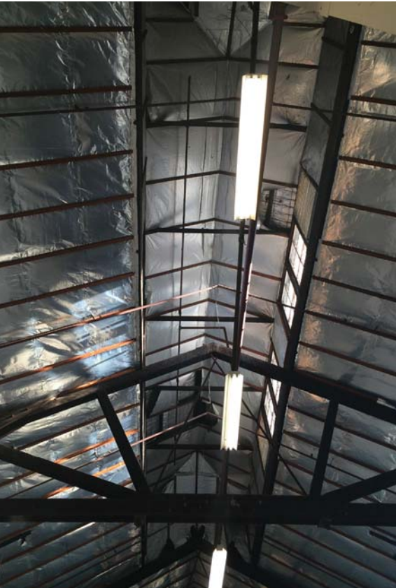
Ceilings, Truss + Lanterns
