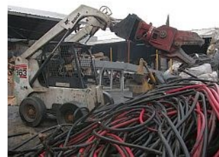
b) Bob Cat with Demolition Shears with Demolition Shears
