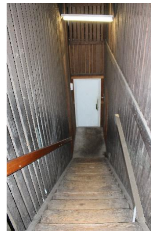
Existing Heritage timber stair
