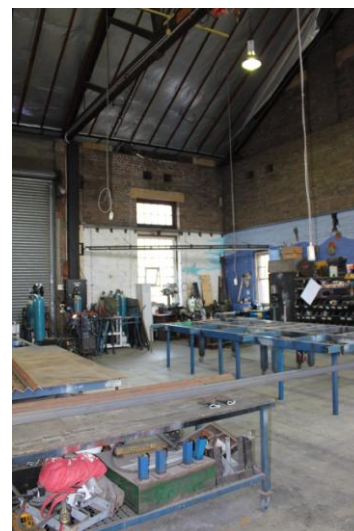
Existing loading area
