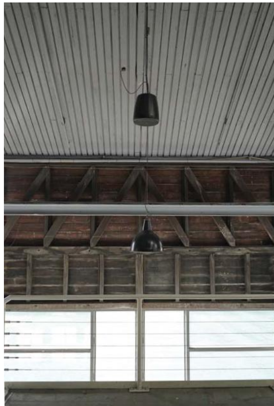
Figure 35: Existing timber batten ceiling
