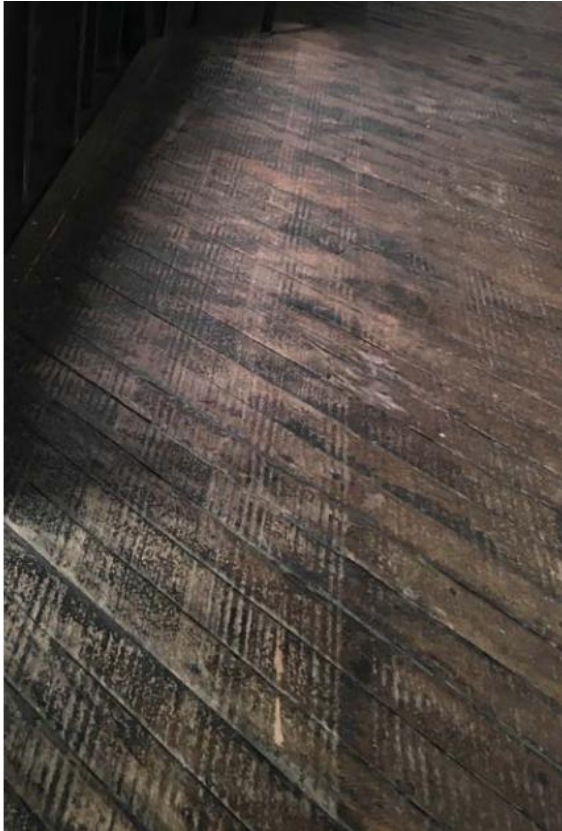
Figure 32: Original Ironbark floorboards
