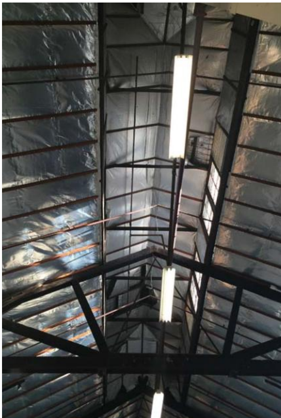
Figure 34: Existing foil ceiling
