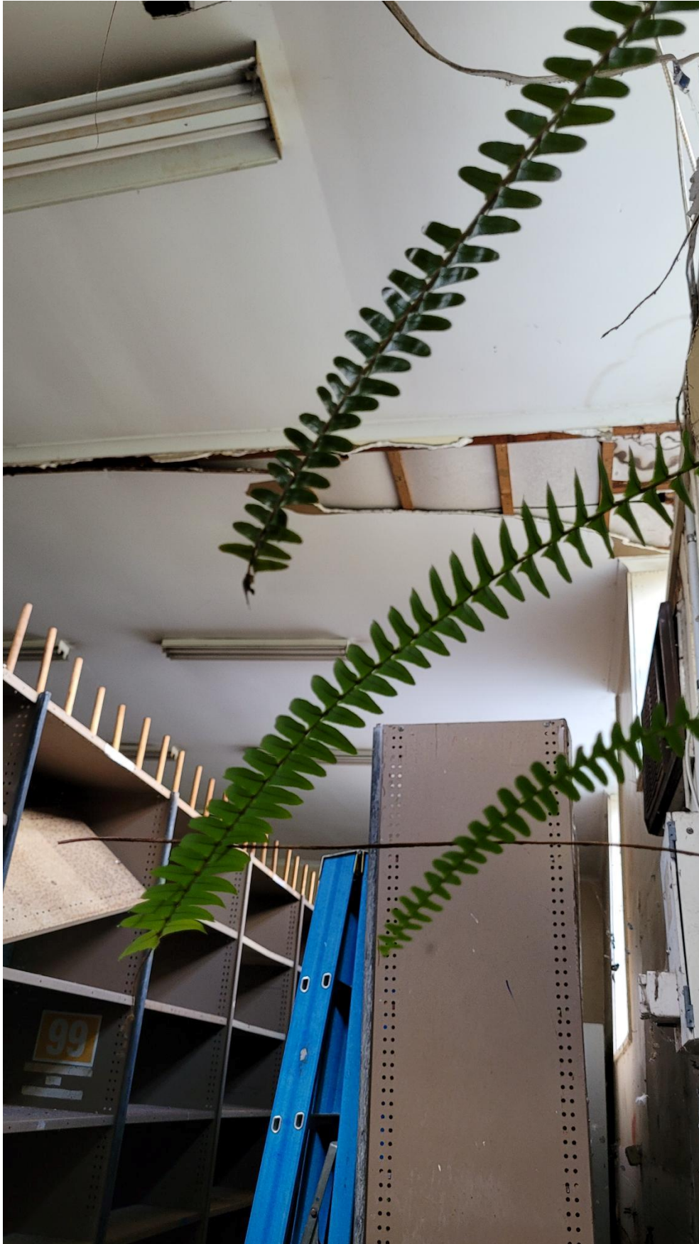
Photo 2: Exposed ceiling cavity in the shed onsite.
