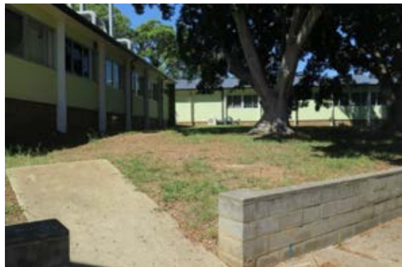
Figure 3.8 View into a courtyard between three c1950 former hospital buildings with a retaining wall visible in the foreground. (Source: GML 2016)
