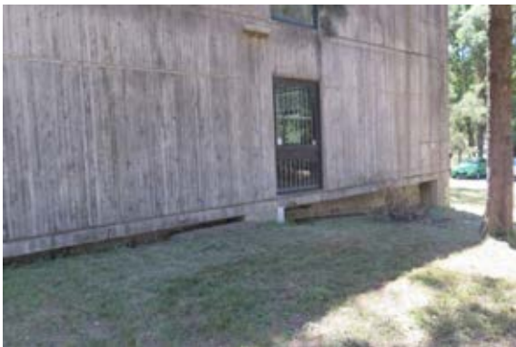
Figure 3.7 View of one side of a formed concrete building at the southwest corner of the study area, showing the likely presence of a basement level. (Source: GML 2016)
