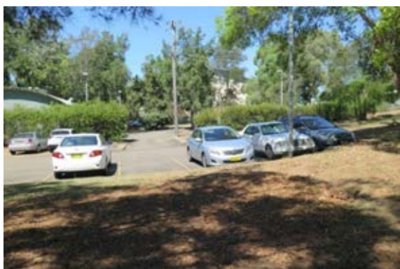
Figure 3.11 View of cutting into the slope of the study area along the southern boundary to construct a car park. (Source: GML 2016)
