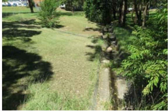
Figure 3.16 View east along the concrete-lined drain extending through the study area. Note that the drain is visibly situated within a minor gully. (Source: GML 2016)
