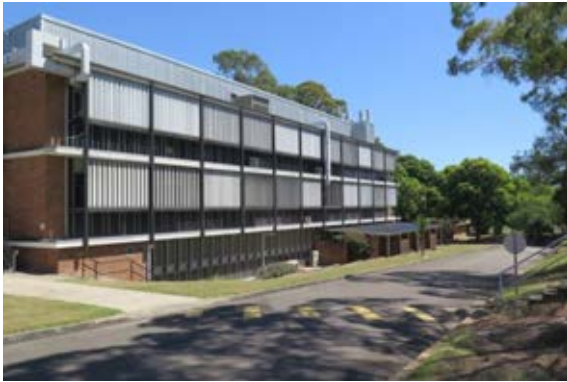
Figure 3.5 View to the west along the northern extent of the large U-shaped building. (Source: GML 2016)
