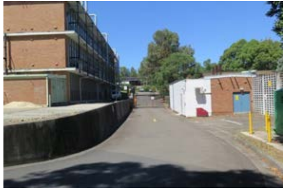
Figure 3.4 View to the east along the southern side of the U-shaped building (left). (Source: GML 2016)
