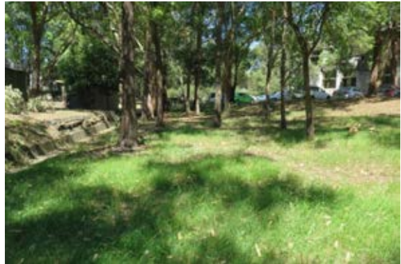
Figure 3.18 View to the southeast showing the concrete-lined canal with green vegetation and trees within a minor gully. (Source: GML 2016)
