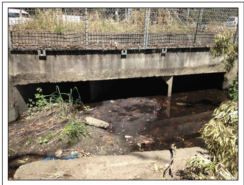
1800 CULVERT APPEARS TO BE THE CULVERT FROM ACROSS THE ROAD.
