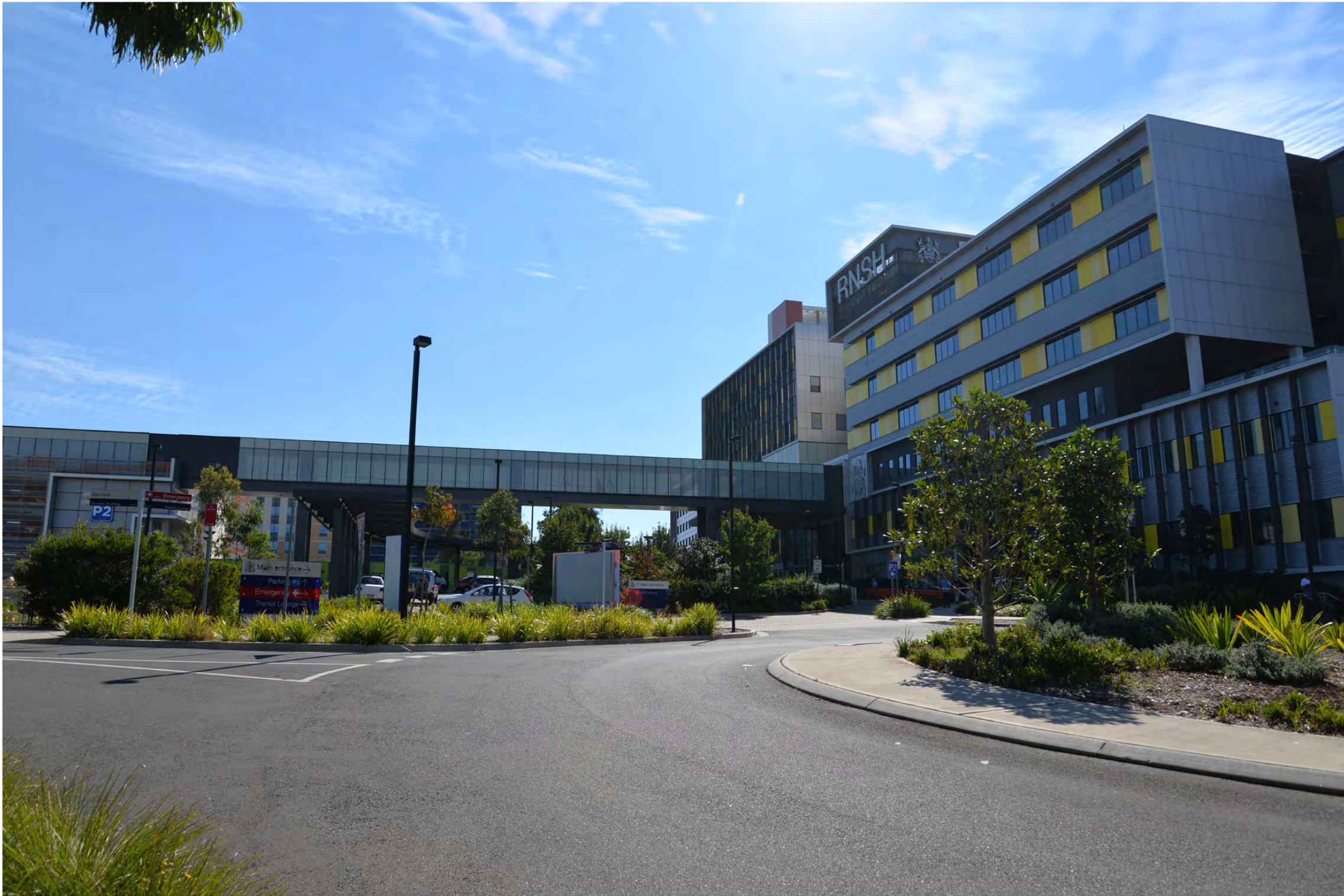
VIEW E, From Reserve Rd (South - West)
