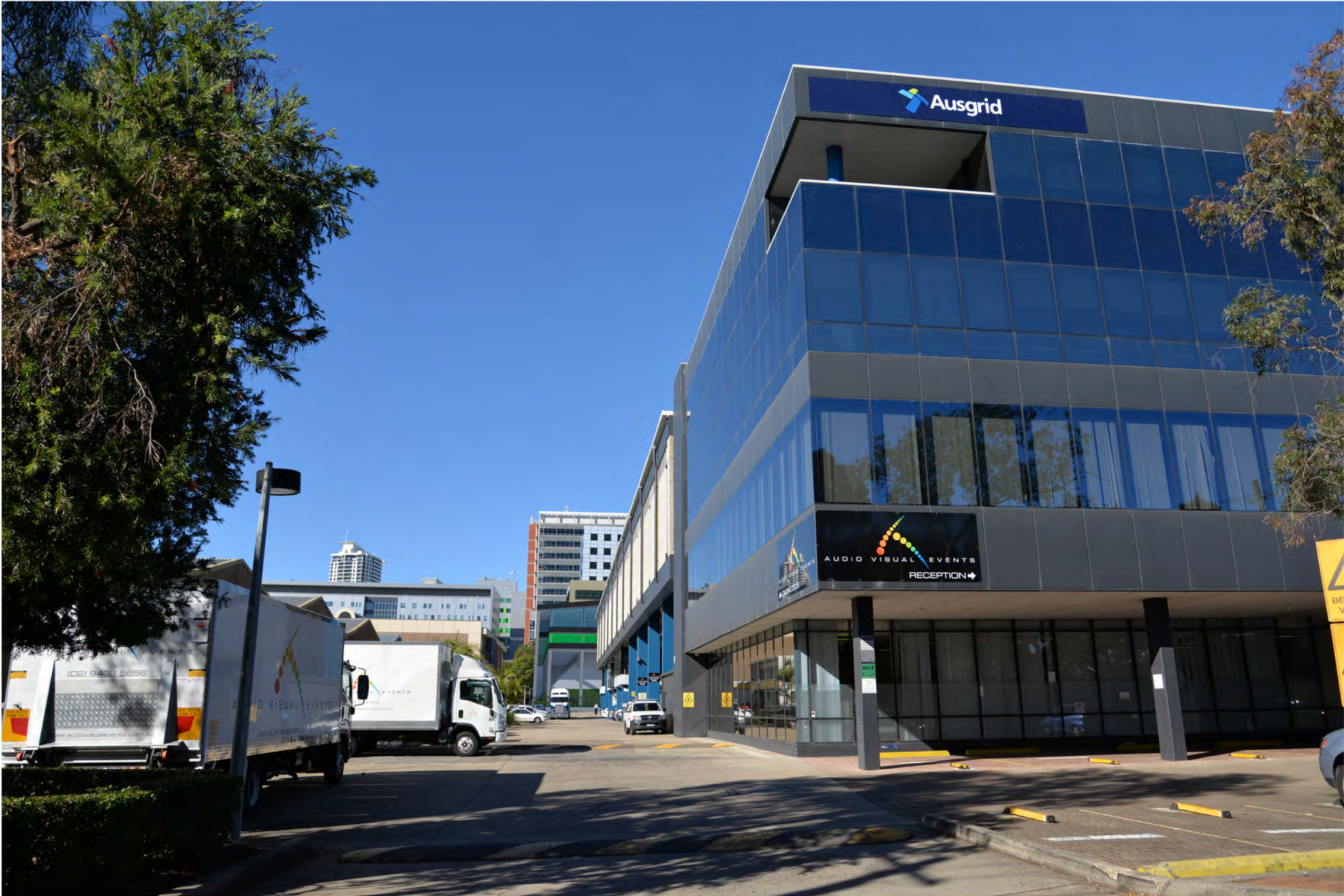
VIEW G, From Frederick St Dexus Warehouse Driveway Entry
