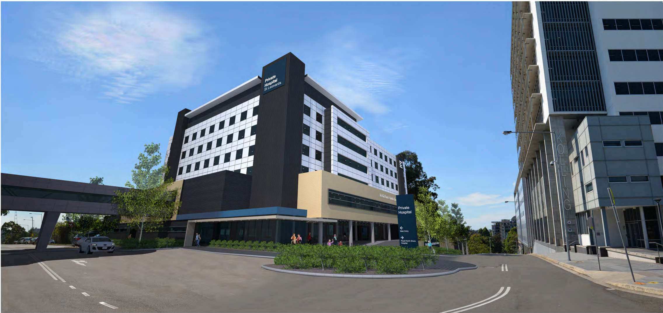
VIEW A, From Intersection Of Reserve Rd & Westbourne St
