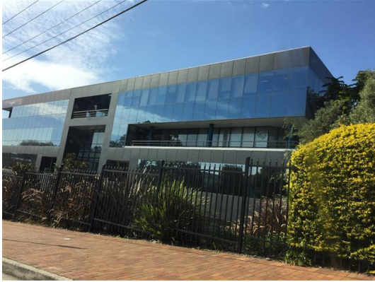
Figure 2.5: 12 Frederick Street (subject site)
