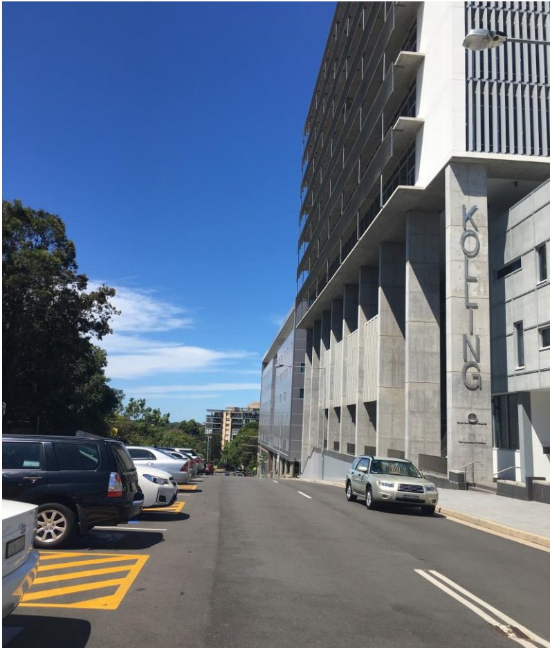
Figure 4: View looking along Westbourne Street, with Kolling Institute to the south of the site
