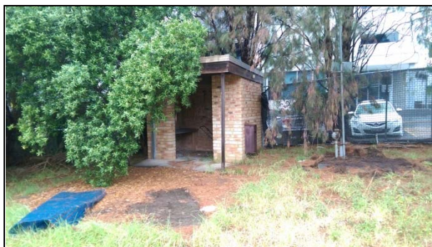
Photo 1: brick structure and underground petroleum storage infrastructure.
