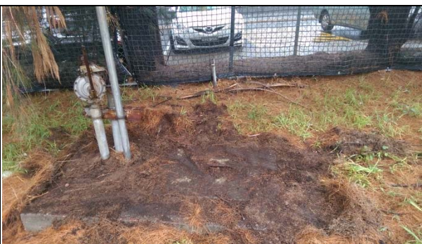
Photo 2: concrete slab with suspected hand pump and vent pipe.
