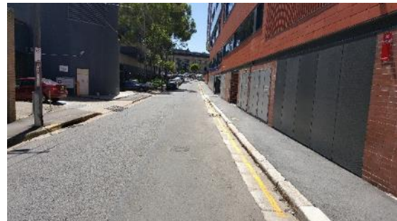
Figure 2.5: Lucas Street (looking east)
