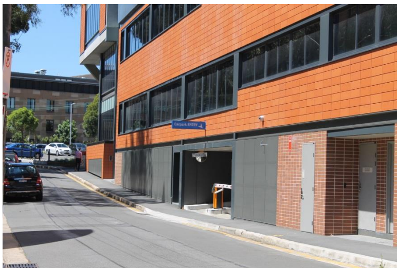
Figure 14 – Car park entry to the Marie Bashir Centre on Lucas Street
