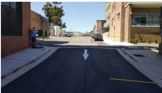
Figure 2.10: Grose Street and New Road (looking south)
