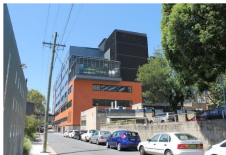
The Marie Bashir Centre viewed from Lucas Street
