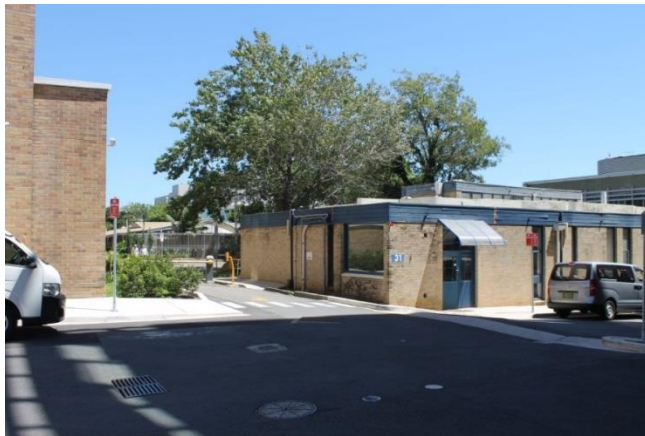
View of the site office and existing car park, viewed for Lucas Street
