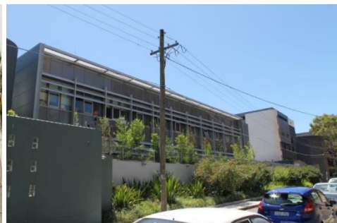
Consulate General building viewed from the eastern end of Lucas Street
