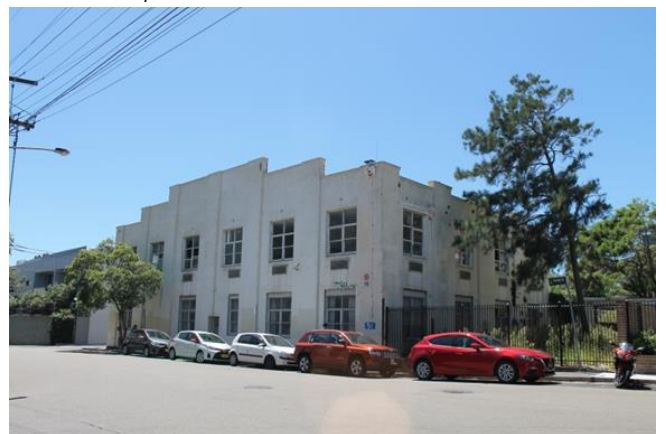
View of two storey building on the Site, viewed from Church Street, looking north east
