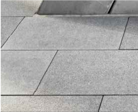
CODE: P1 + P1A DESCRIPTION: STONE PAVING ON GRADE/STRUCTURE SIZE: 600x400x40mm COLOUR: SESAME GREY
