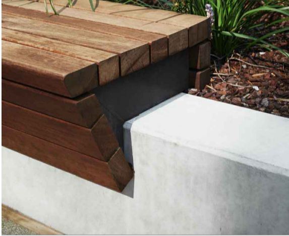
CODE: FU1 DESCRIPTION: CUSTOM TIMBER SEATING TO WALL COLOUR: CLASS 2 AND STAINED HARDWOOD
