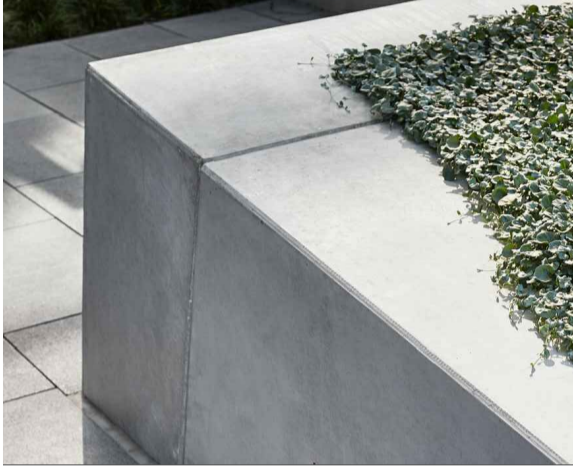
CODE: W1 DESCRIPTION: CONCRETE PLANTER WALL FINISH: CLASS 2
