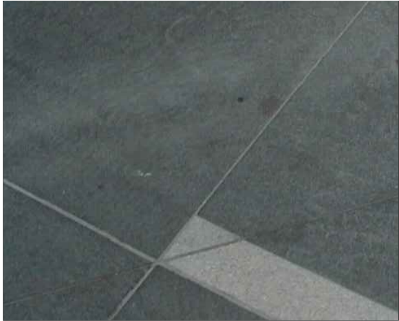
CODE: P2 DESCRIPTION:STONE BANDING PAVING SIZE: 600x400x40mm FINISH: RAVEN BLACK
