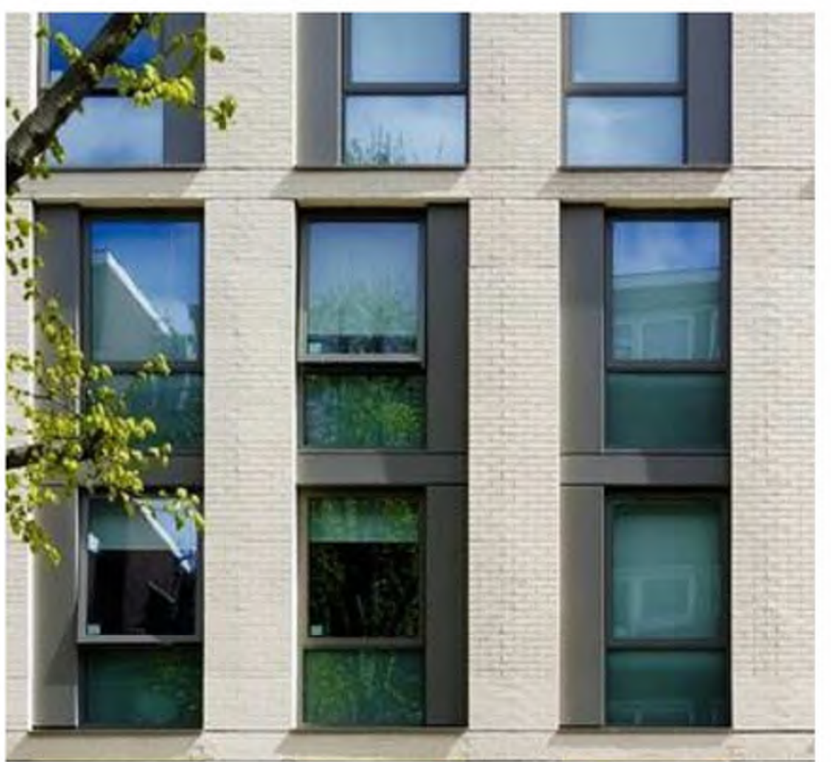
③ DARK ANODISED ALUMINIUM WINDOW FRAMES WITH FROSTED LOWER PANELS
