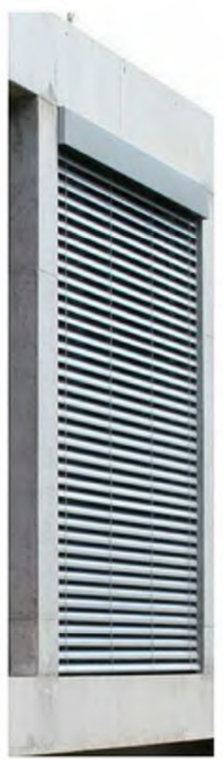
⑥ EXTERNAL LOUVRES BLINDS TO NORTHERN FACADE OF STAIRS
