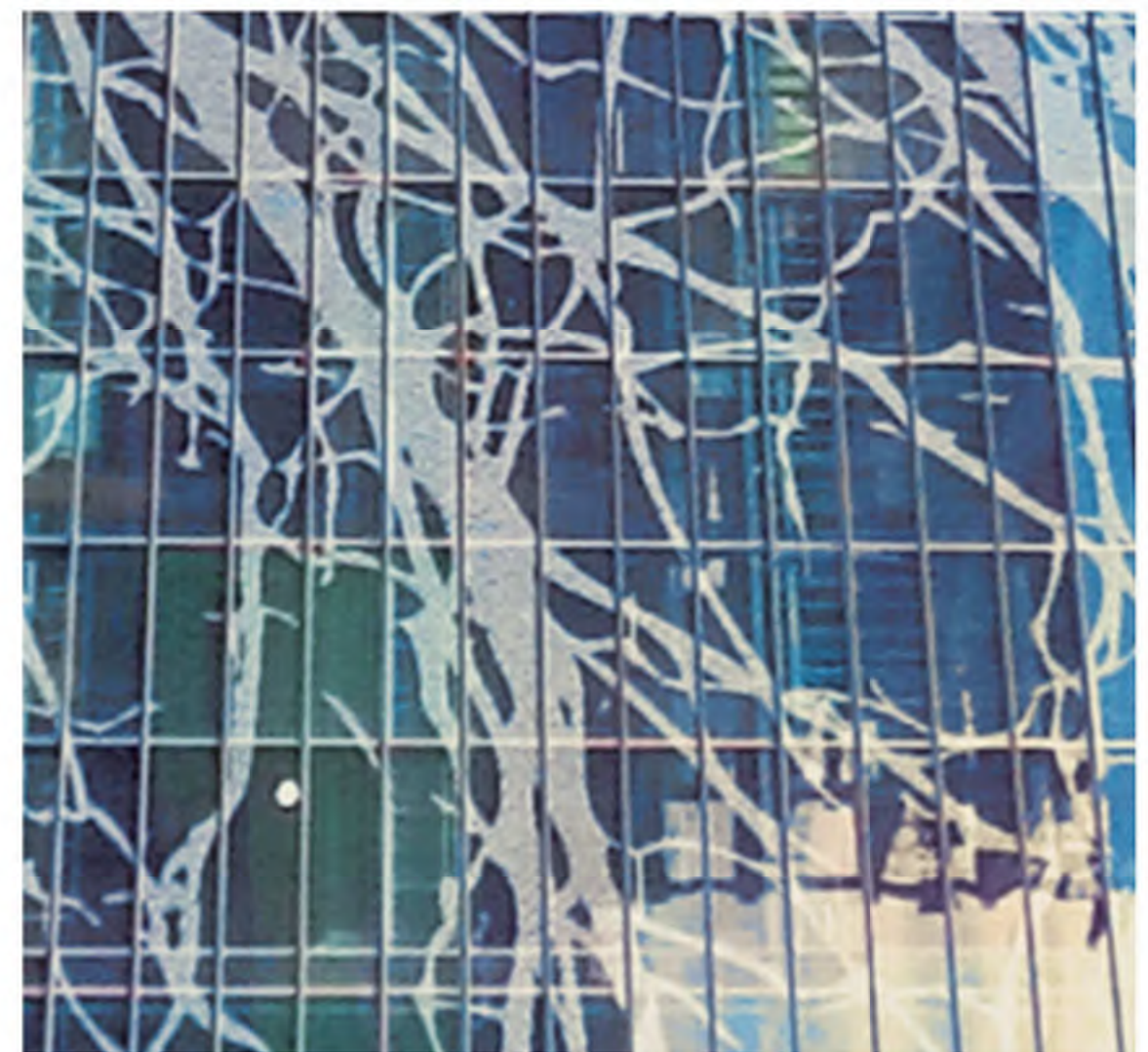
② GLASS CURTAIN WALL WITH FROSTED IMAGERY
