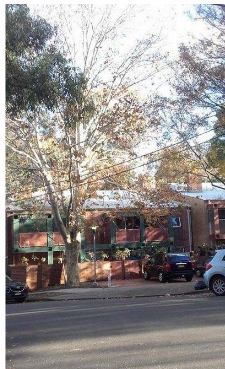
Figure 2.27 Newtown Darlington Suites facing west from the corner of Darlington Lane and Golden Grove Street
