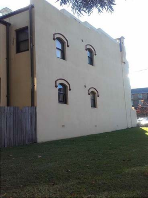
Figure 2.7 Eastern facade of 86 Darlington Road looking west from the corner of Darlington Road and Codrington Street
