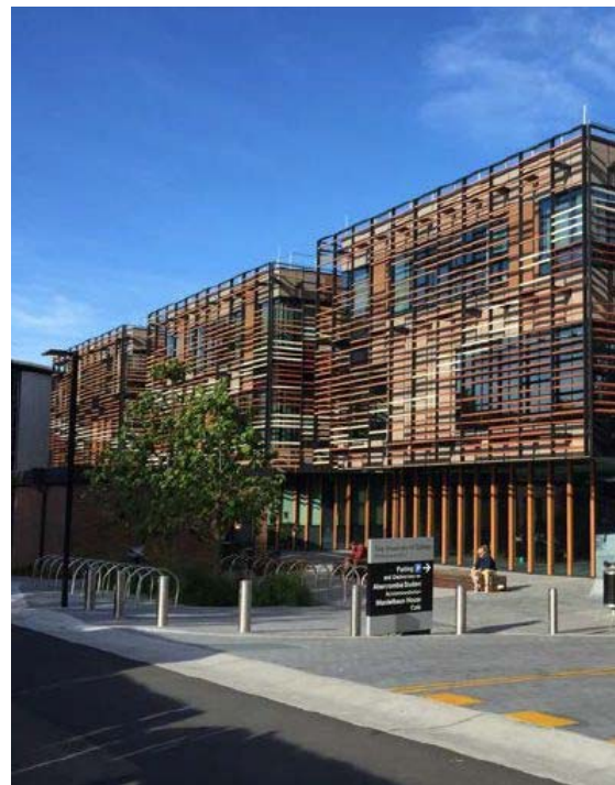
Figure 2.23 Abercrombie Business School ground floor learning area looking east from Darlington Lane
