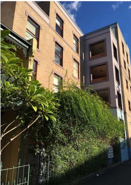
Figure 2.9 Darlington House looking west towards Golden Grove Street
