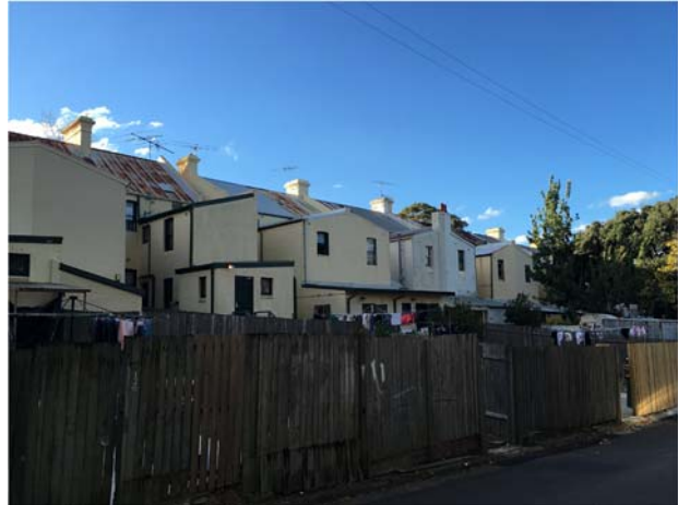
Figure 2.12 Rear yards of Darlington Road Terraces from Darlington Lane facing north
