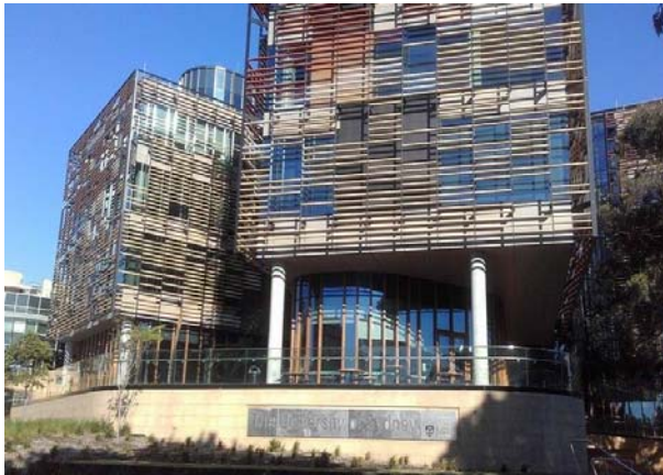
Figure 2.20 Abercrombie Business School facing north-west from the corner of Darlington Road and Abercrombie Street
