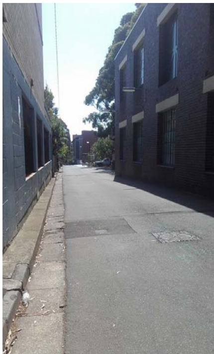
Figure 2.22 Darlington Lane facing east towards Codrington Street. IXL Garage located on the southern side of Darlington Lane
