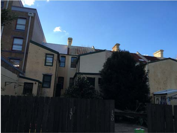
Figure 2.11 Rear yards of Darlington Road Terraces from Darlington Lane facing north
