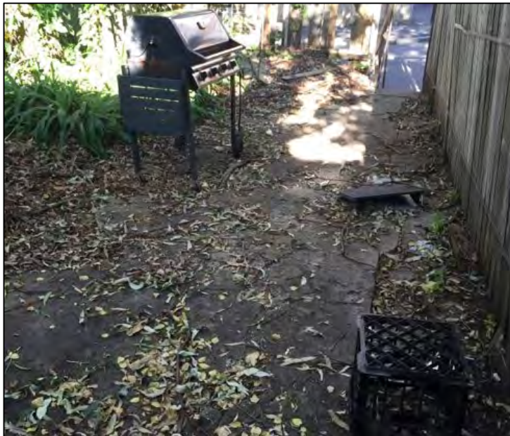
Figure 28: The old concrete paths located with the TPZ of tree 11 that require hand removal or machine removal with Arborist supervision. . Source Austin 27/05/2016
