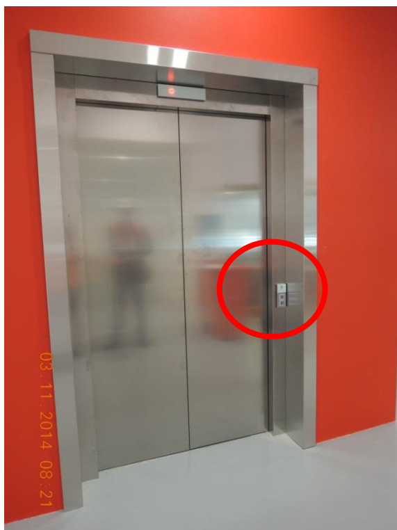
Figure 4 image of non-compliant lift call button installation
